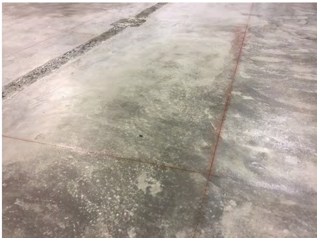
Expansion joint lines
