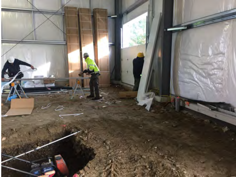
View of Frommelt building mechanical doors
