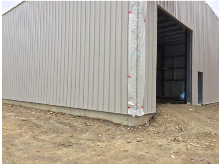
View of temporary trim on wall corner
