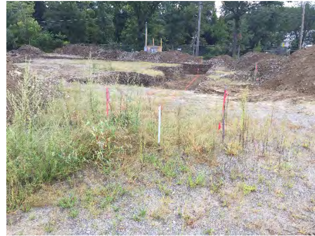
View of foundation hole
