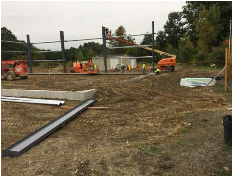
View building erection
