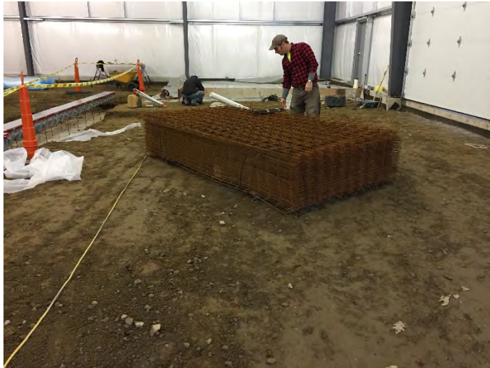
Samson unpacking rebar mesh
