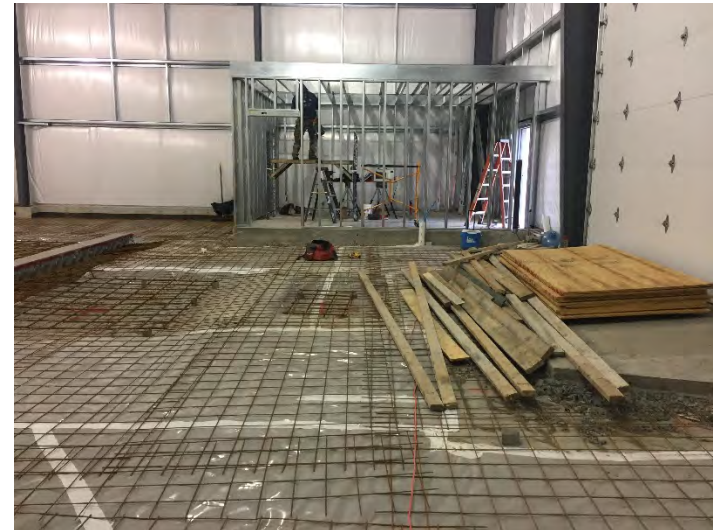
View office framing
