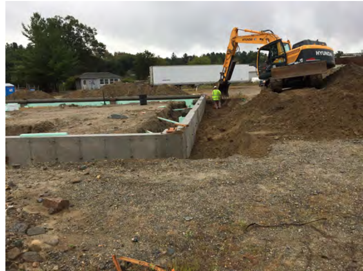
View of Nashoba beginning backfill and compaction
