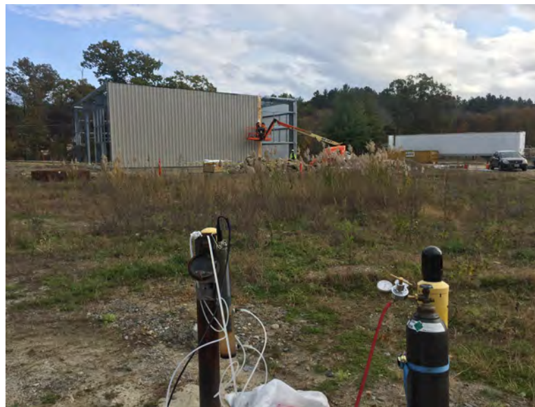
View of insulation/panels being placed
