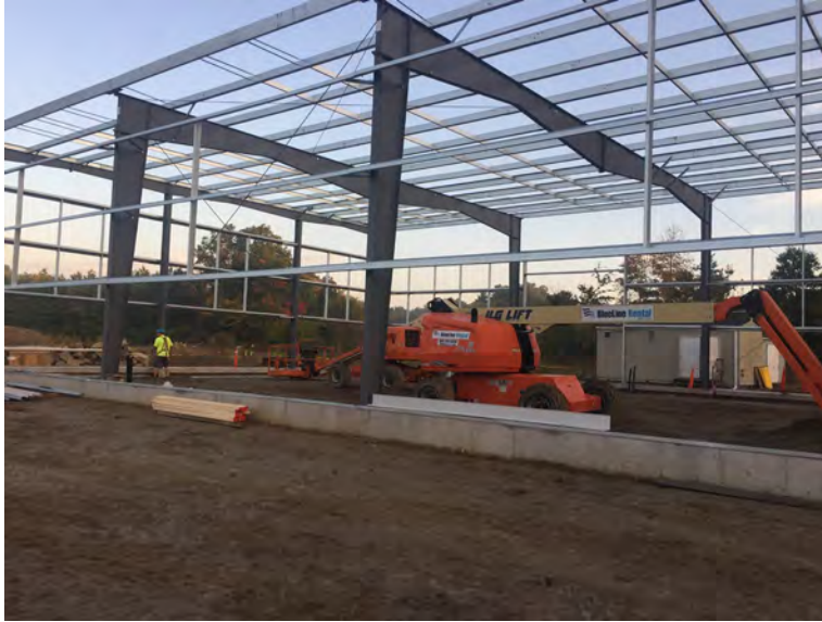
View of building roof progress
