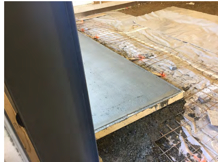
View of Concrete in ramp form
