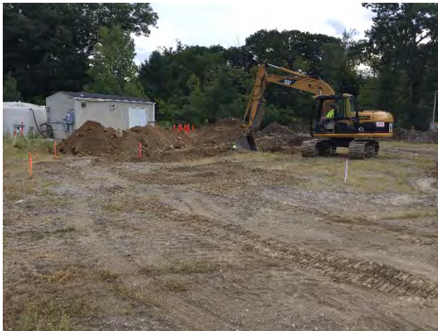
Working on digging the foundation
