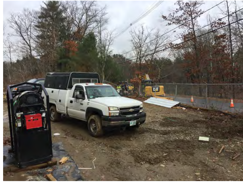
View of Onyx working on public water line
