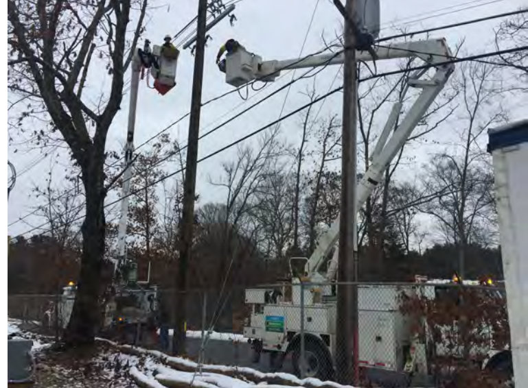
View of Eversource working on new electrical pole
