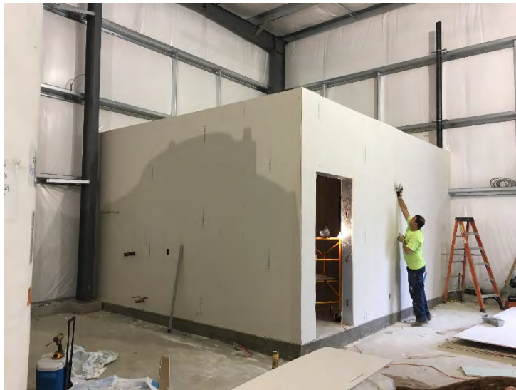
View of drywall on office
