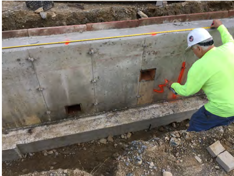
View of bathroom pipe sleeves
