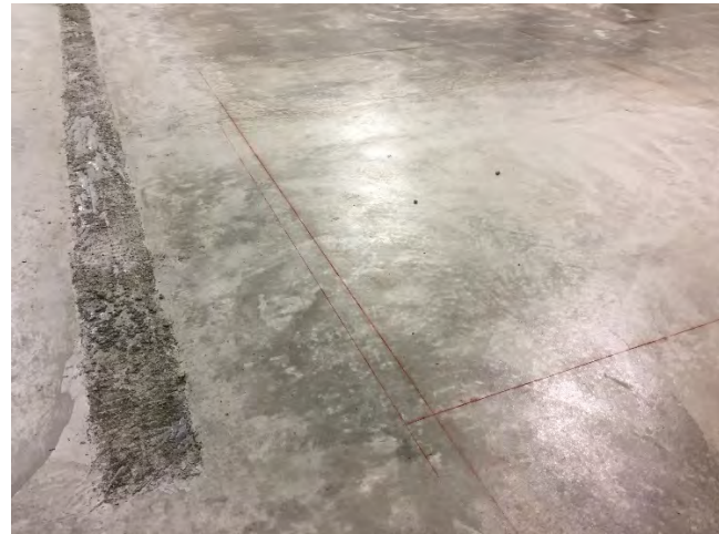
Expansion joint lines
