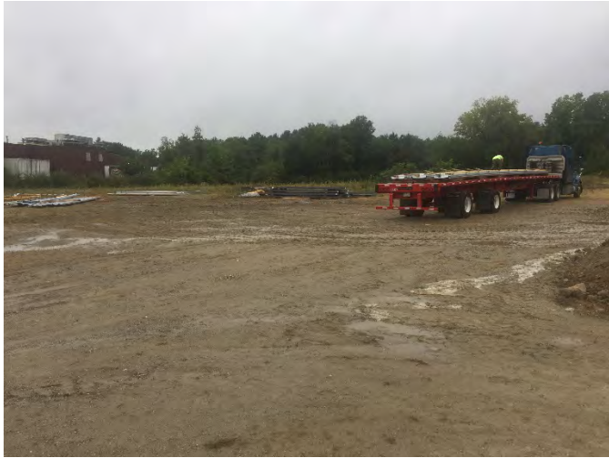
View of Building Delivery
