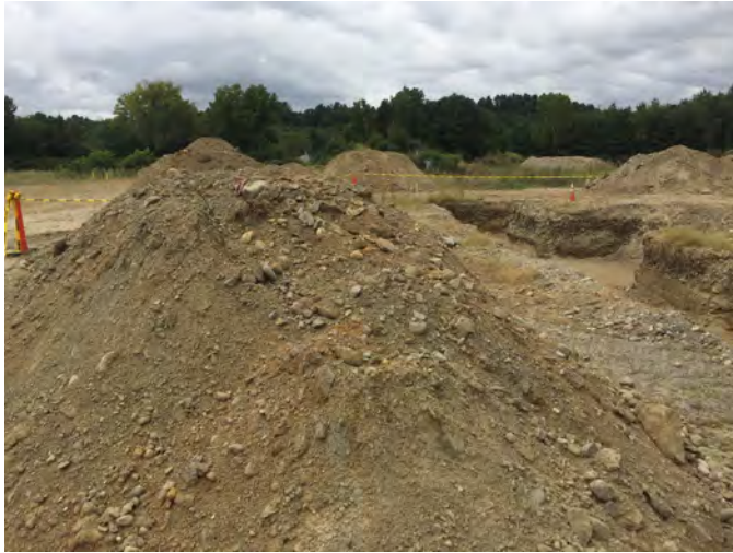
View of foundation hole
