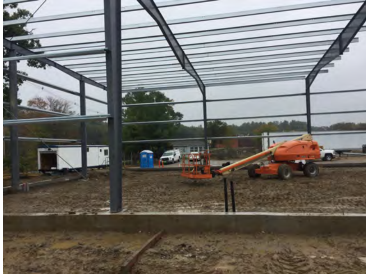
View builders adding roof panels
