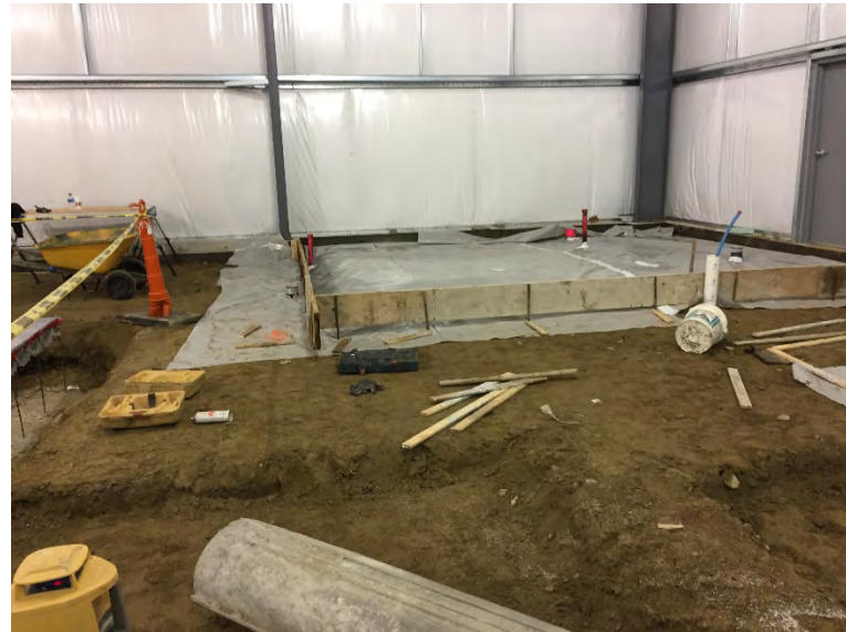
Framing of Office foundation
