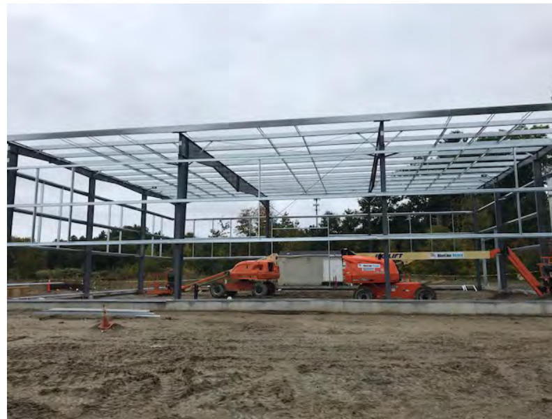
View of building progress
