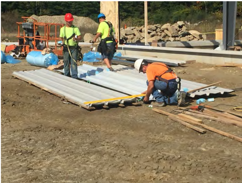
Setting up wall panels with blue foam separators
