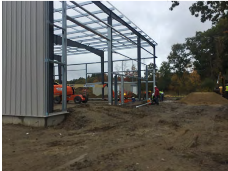
View of prep work for more panels
