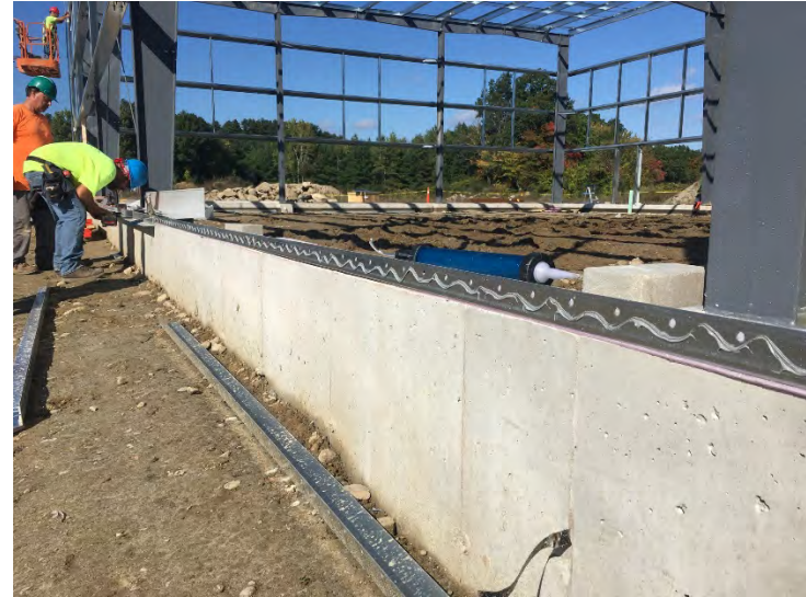
View of caulking trim pieces
