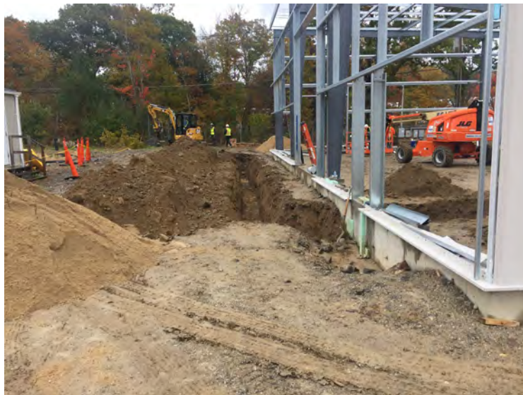
View of trench for domestic water line
