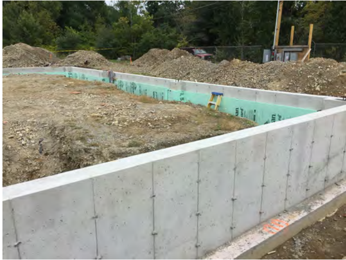
View of Foundation with insulation
