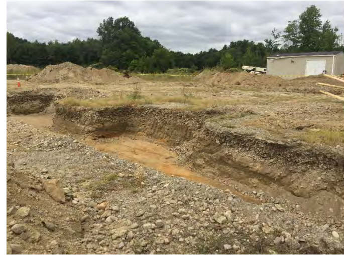
View of foundation hole
