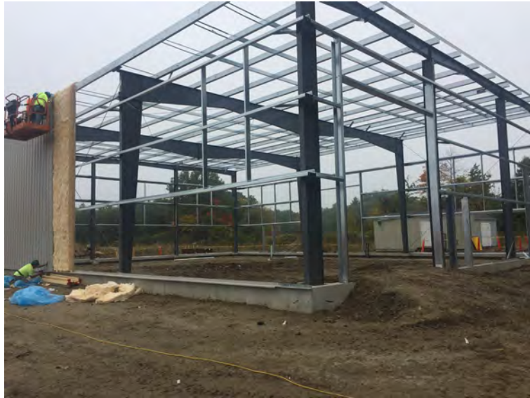
View of insulation, panel wall
