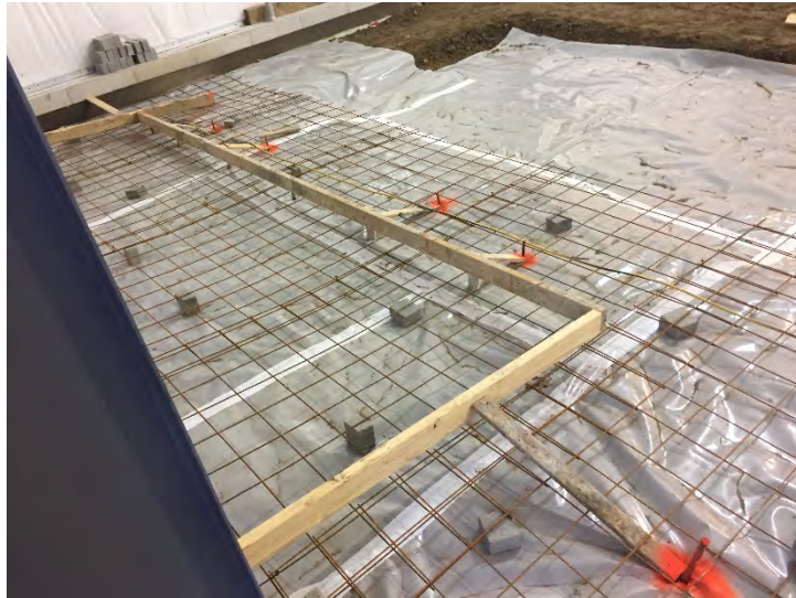
View of fully framed concrete ramp
