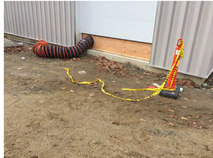
View of how temporary heat will enter building
