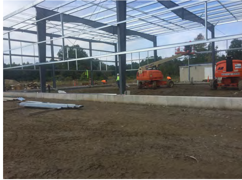
View of builders adding wall supports
