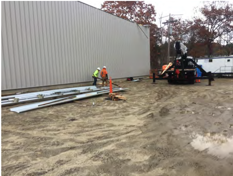
Crew working on identifying building parts
