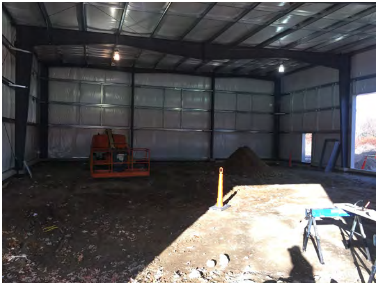
View of inside building with temporary lights
