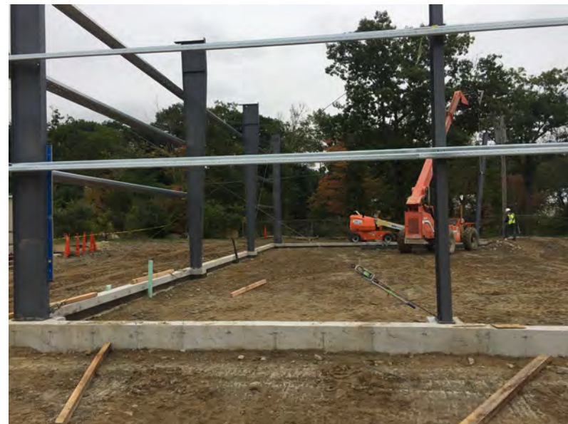
View of steel and support cables
