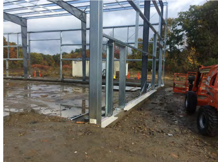
View of walls to be completed
