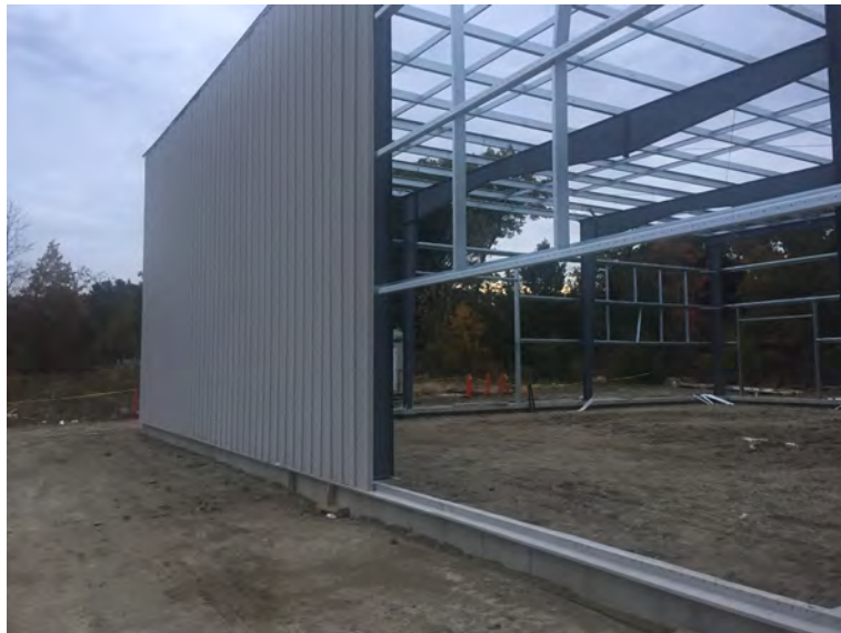
View of insulation, panel wall
