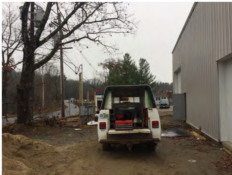
View of Frommelt building mechanical doors
