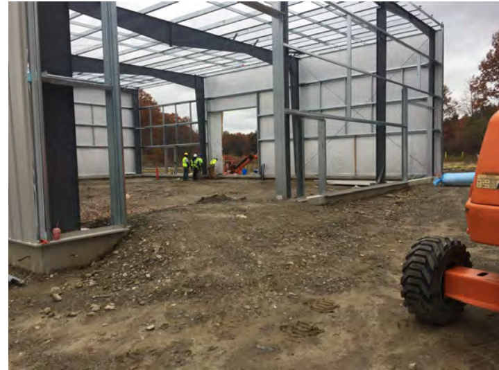
Crew working on north wall panels
