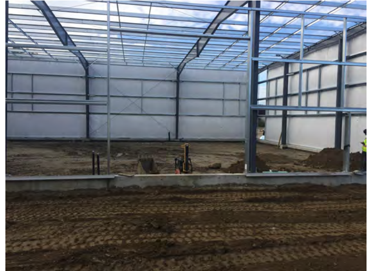
View of completed section of the wall
