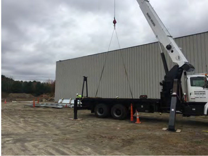
Regional Builders crane to work on roof
