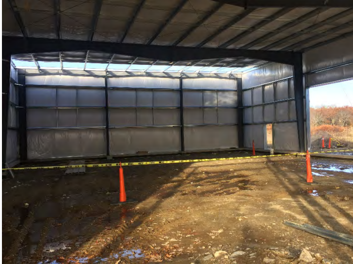
View of roof progress
