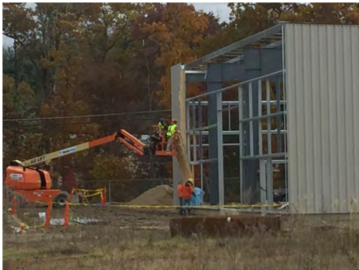
View of panels being placed
