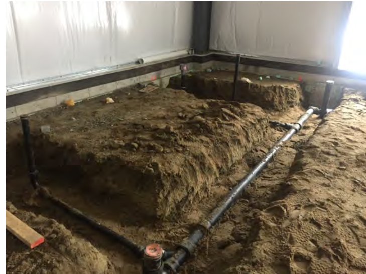
Underground plumbing for building office
