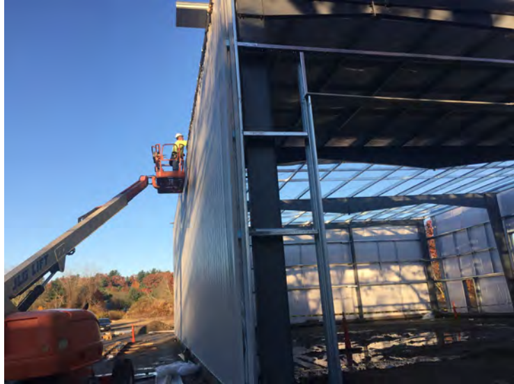
Crew working on roof
