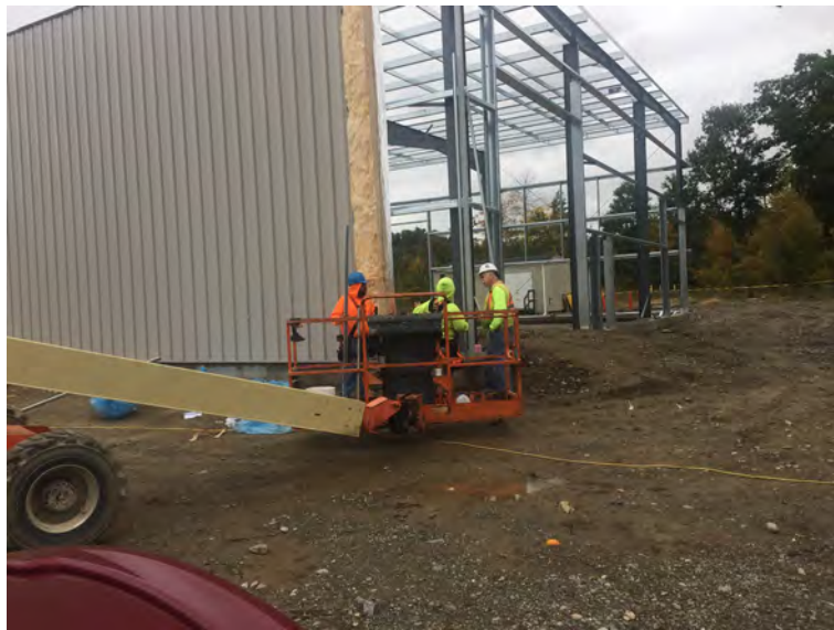
View of measurements before placing insulation/panel
