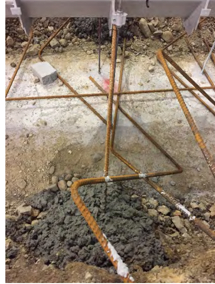
View of trench drain supports
