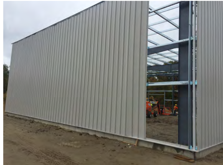
View of completed section of the wall
