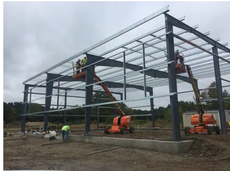
View of builders continuing roof crossbeams
