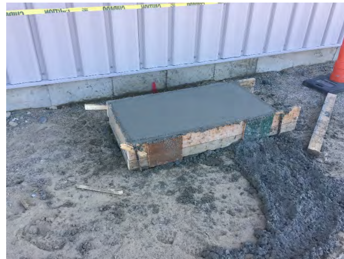
View of Concrete slab pour for air compressor
