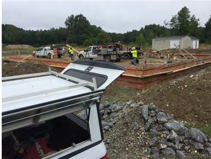
View of Samson finishing wall forms
