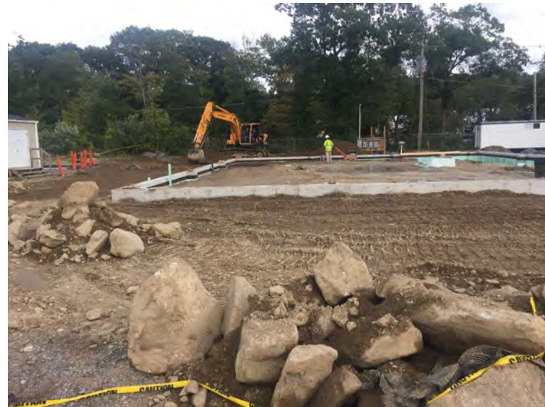
View of backfilled and compacted areas
