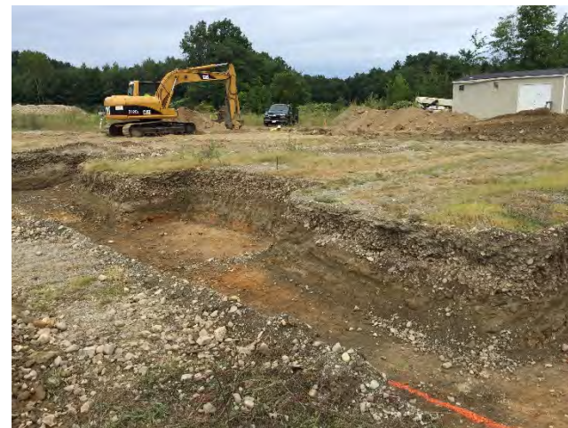
Working on digging the foundation
