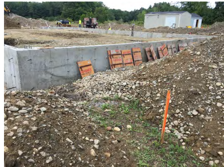
View of Complete foundation without forms
