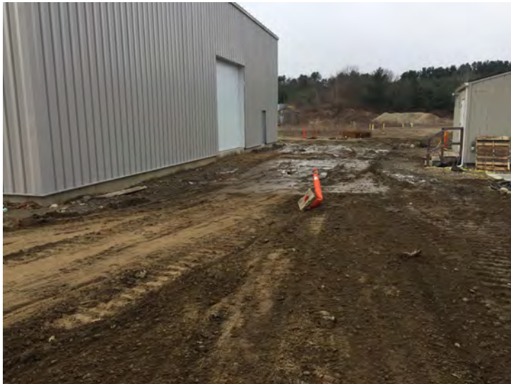
View of North Mechanical door
