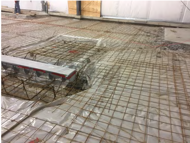
View of wire mesh
