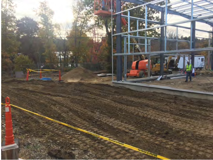
View of filled in water line trench
