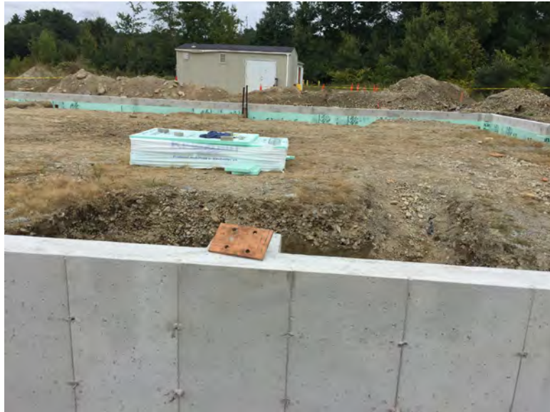
View of Foundation with insulation
