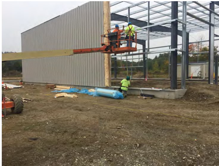
View of measurements before placing insulation/panel
