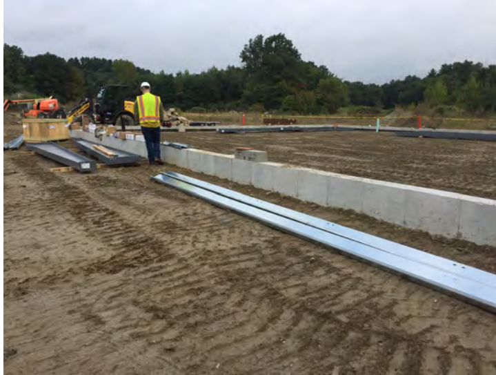
View foundation w/ layed out parts
