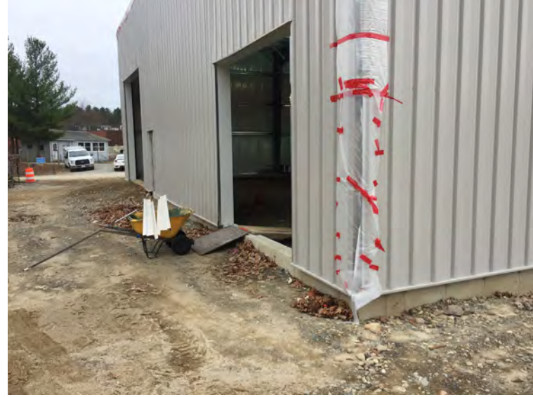
View of completed east wall, and initial trim
