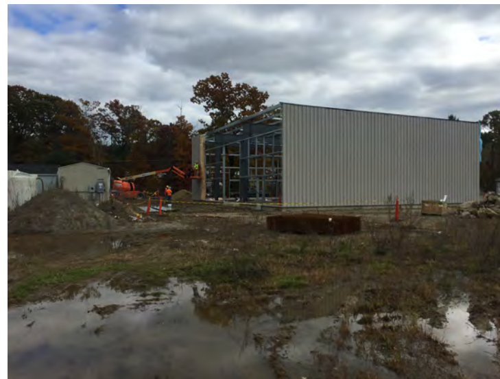
View of panels being placed
