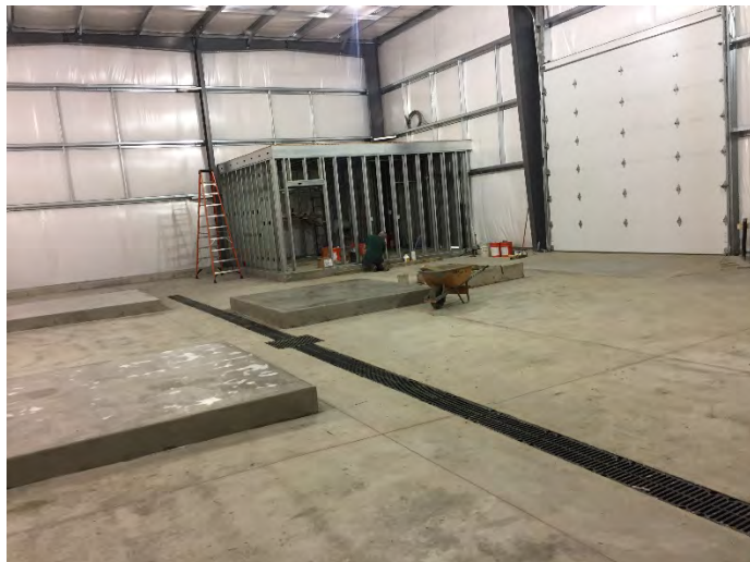
View of electrical work in building office
