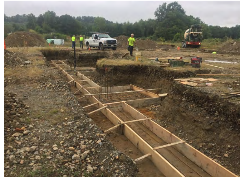
View of Foundation forms with Rebar
