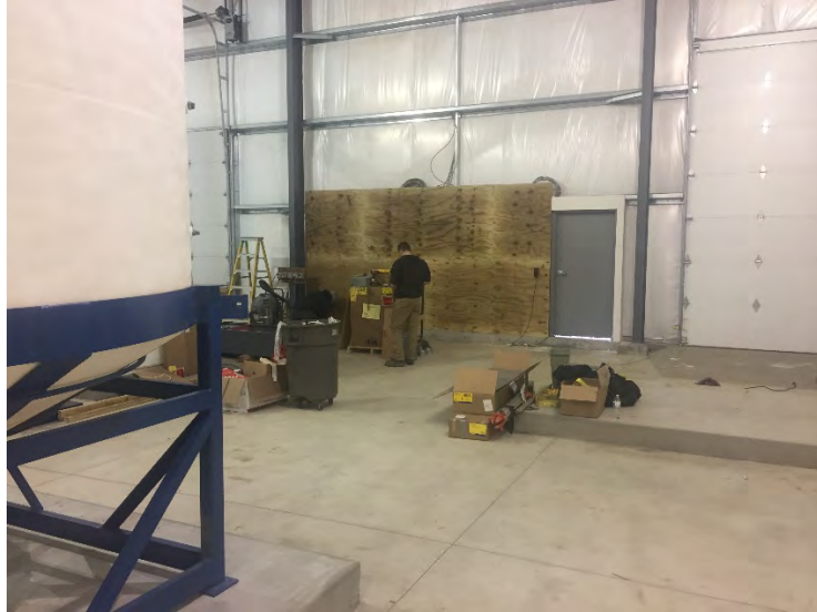
View of electrical panel installation
