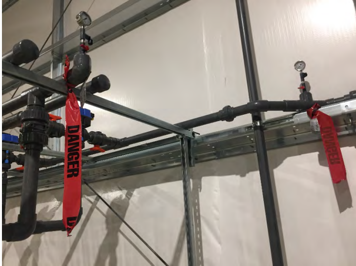
View of treatment system progress
