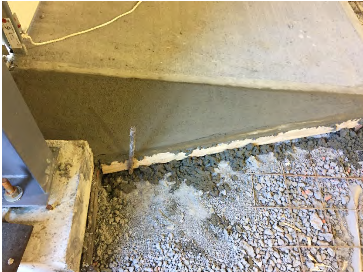
View of Concrete in ramp form
