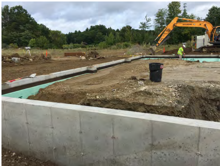
View of Nashoba beginning backfill and compaction
