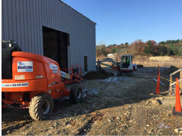
View of exterior exaction for plumbing
