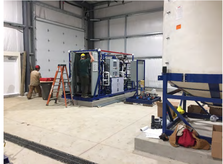
View of electrician wiring Vanox unit
