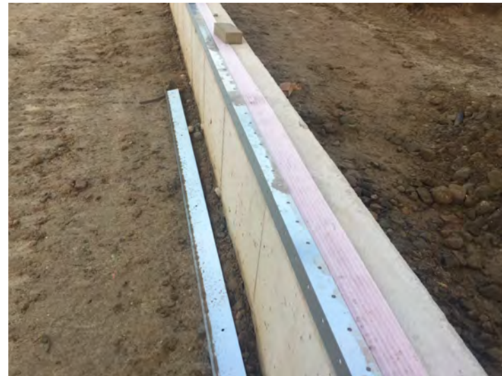
View of trim progress
