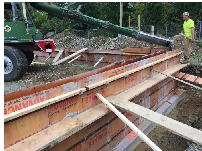
View of concrete being poured into foundation wall forms
