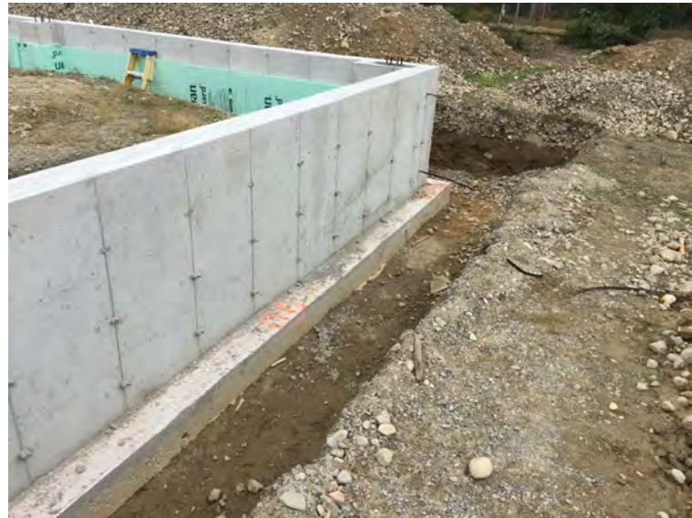
View of Foundation with insulation
