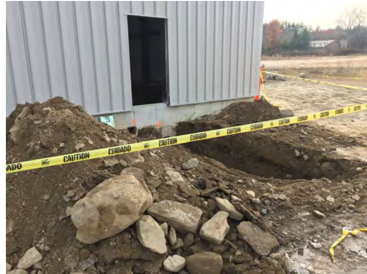
View of exterior excavation in roped off area
