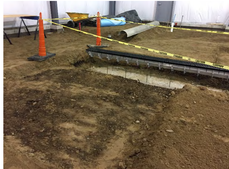
View of Grading work inside building
