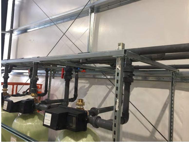
View of continued additions to treatment system
