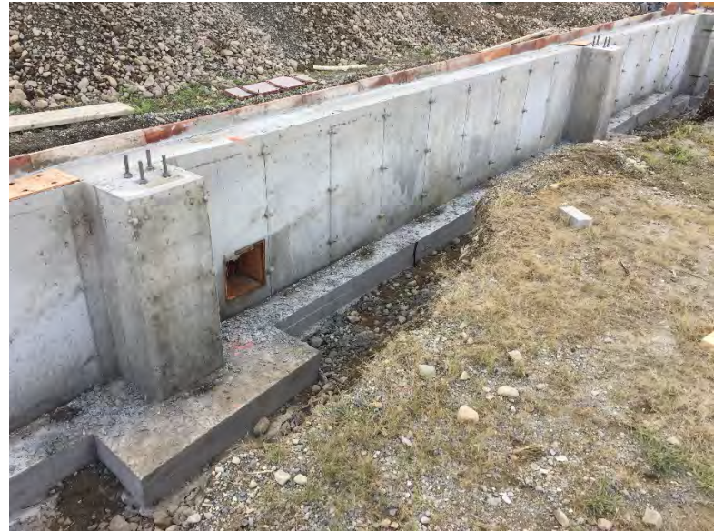
View of foundation wall out of forms
