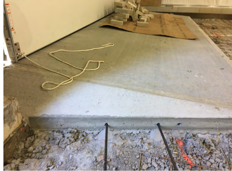
View of slab pore equipment
