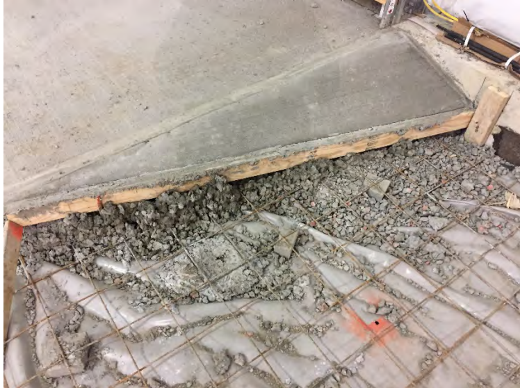
View of cured ramp sides
