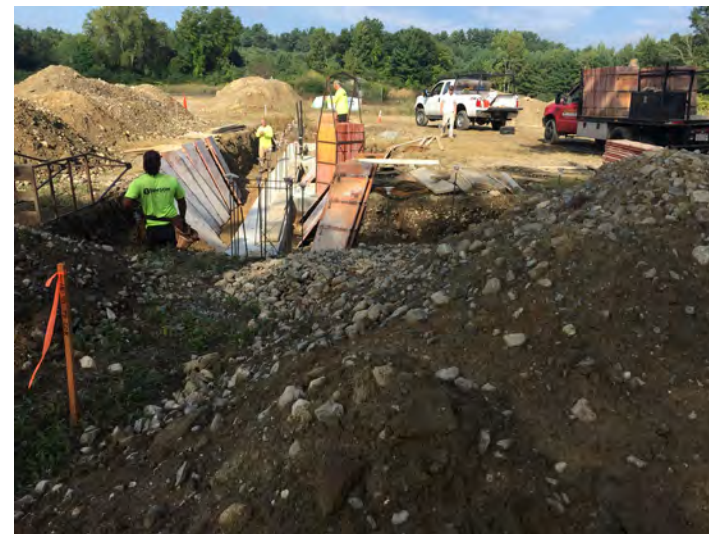
Samson setting up concrete wall forms
