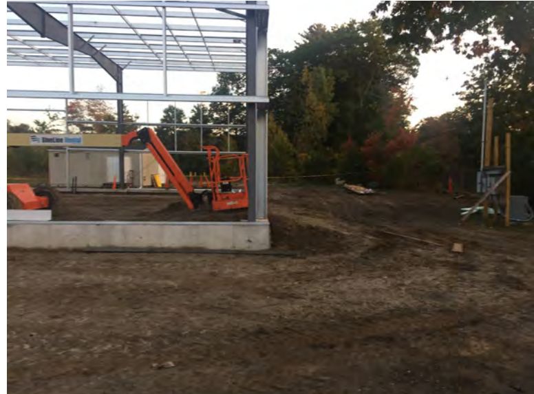
View of building progress
