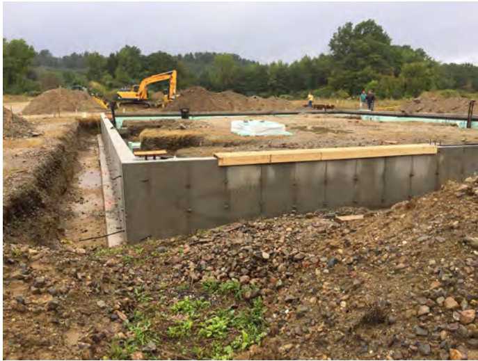
View contractors planning backfill
