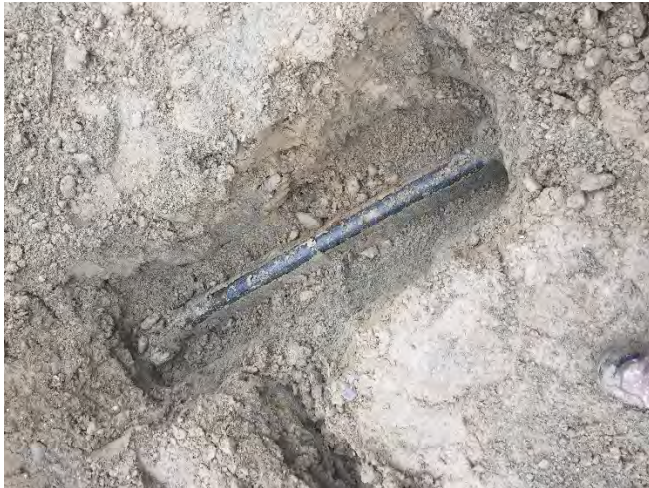
View of existing water pipe
