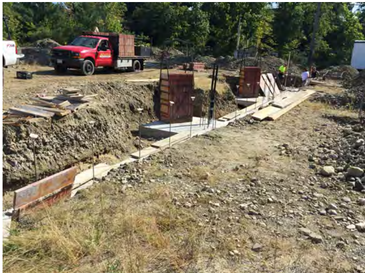
Samson setting up concrete wall forms
