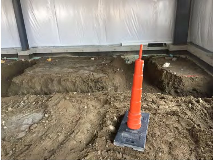
View of indoor plumbing excavation
