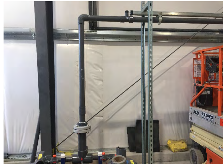
View of continued additions to treatment system
