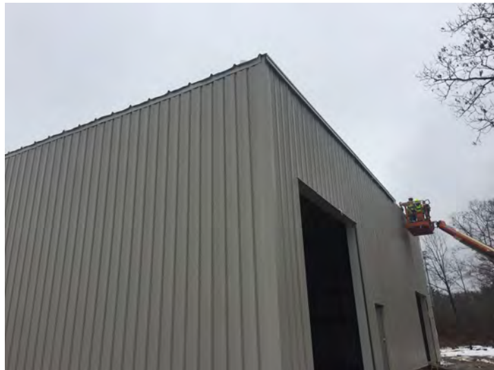
View of trim pieces being placed
