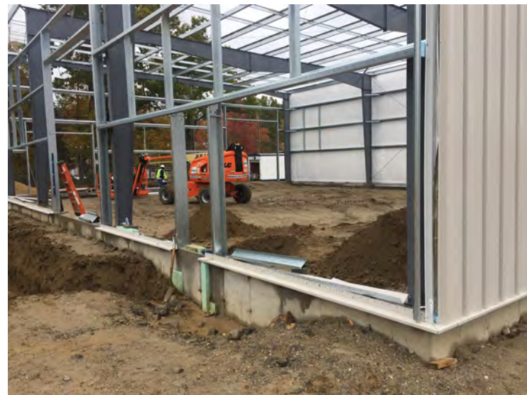
View of side wall prep for panels
