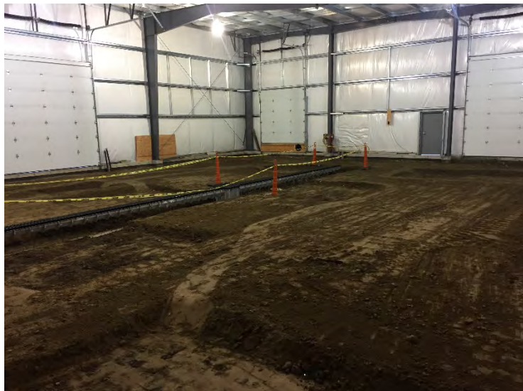
View of completed grading work
