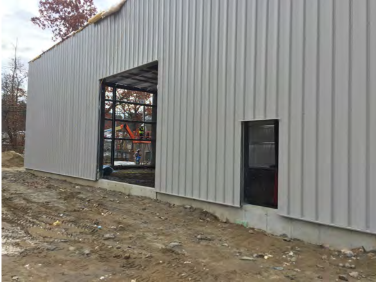
View construction of east wall panels
