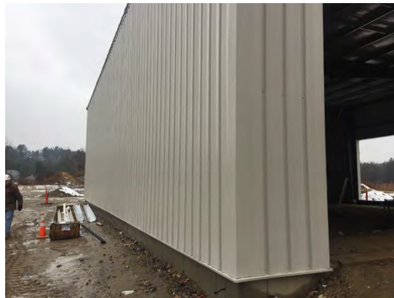
View of trim pieces being placed
