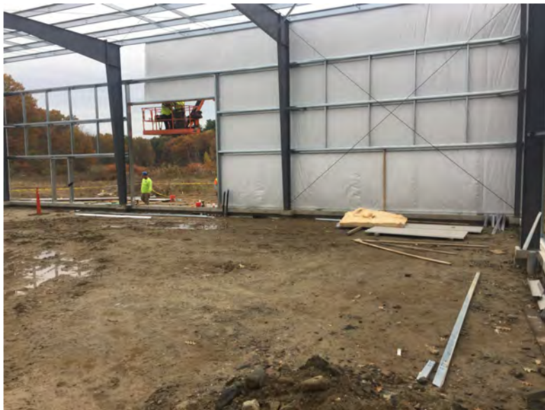
View of panels being placed
