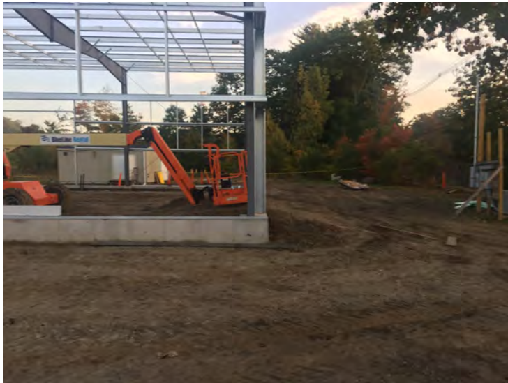
View of building progress
