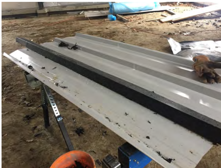
View trim inside being prepared
