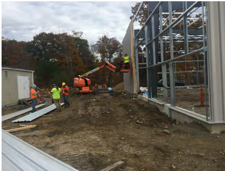
View of panels being placed
