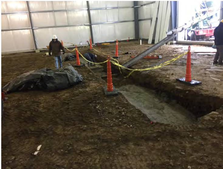
View of Samson Pouring concrete
