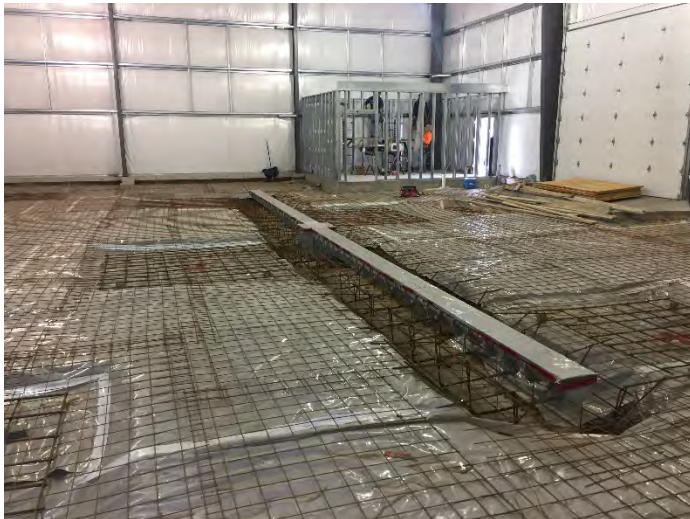
View office framing
