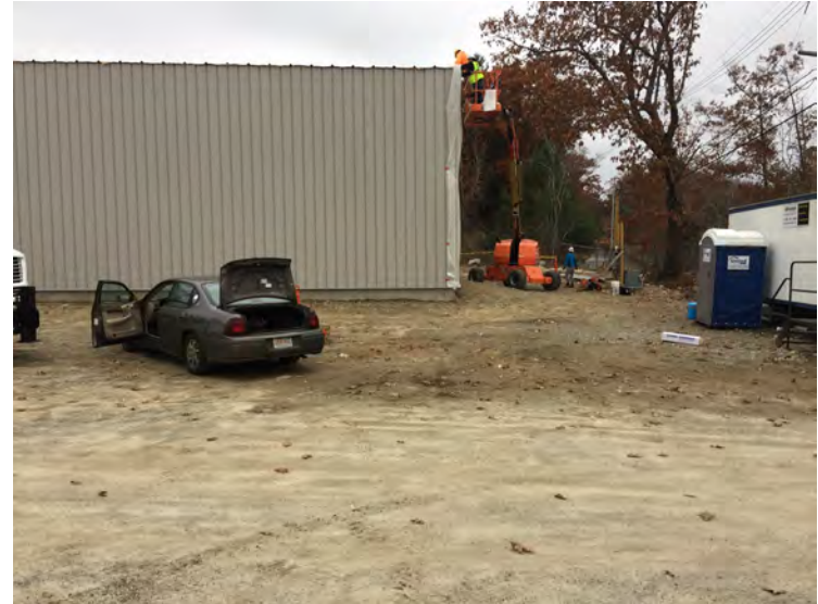
View construction of east wall panels
