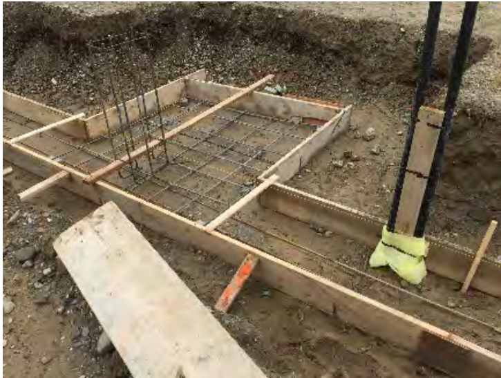
View of 4' footing with rebar setup
