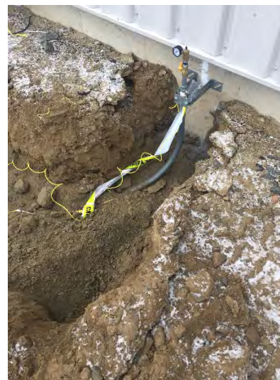
View of trench from propane tank to building
