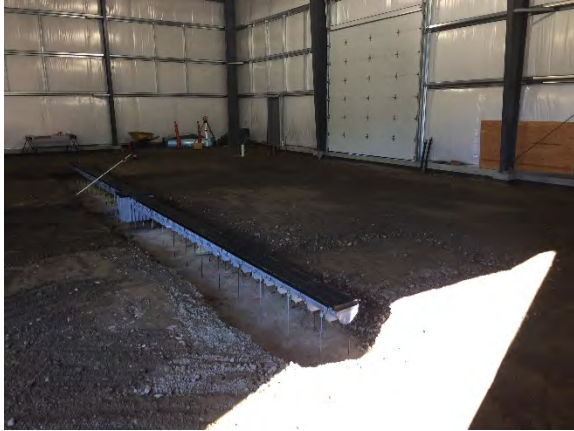
View of Grading work inside building
