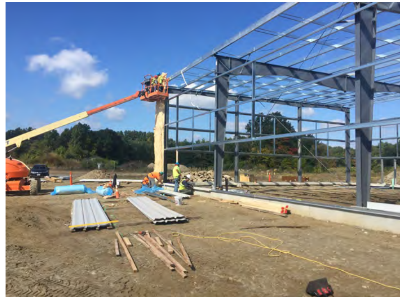
Placings of insulation and wall panels
