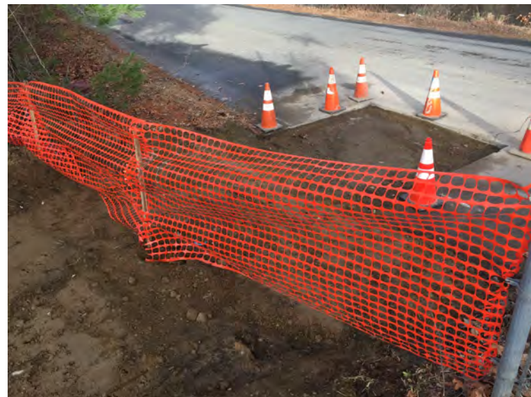
View of Onyx's protection of site work
