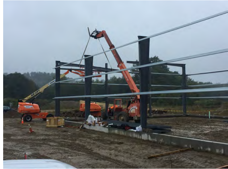
View builders starting roof steel
