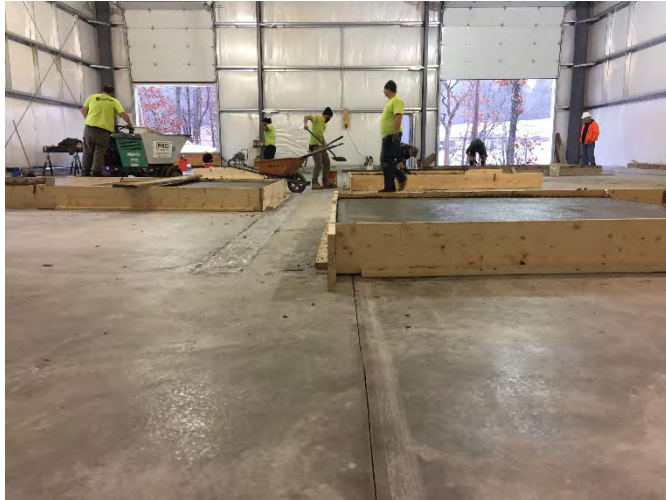
View of riser pad filled
