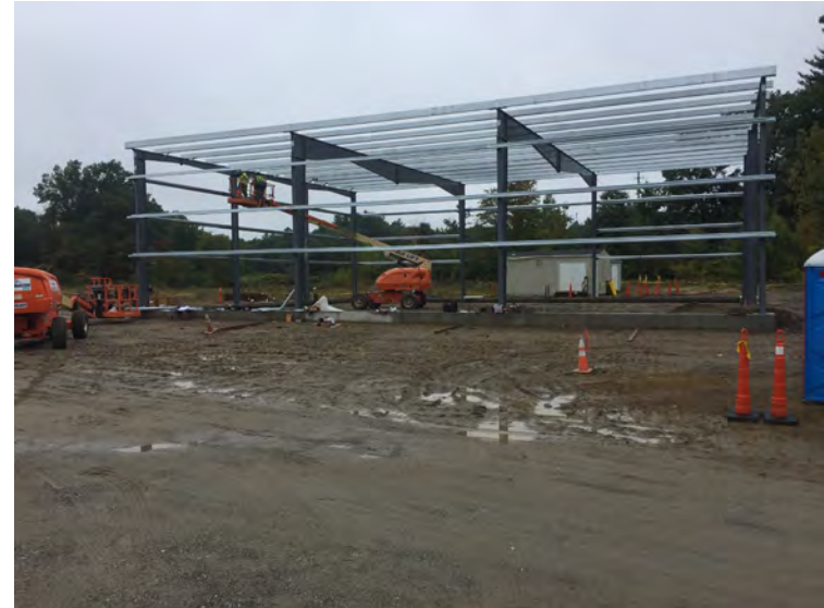
View of builders adding roof supports
