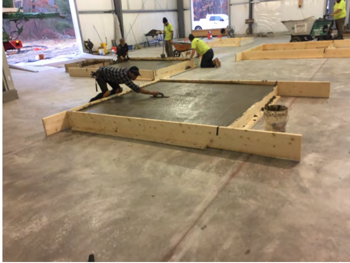
View of riser pad filled
