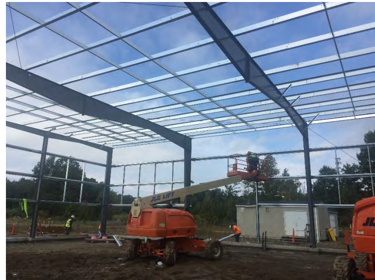
View of builders adding wall supports
