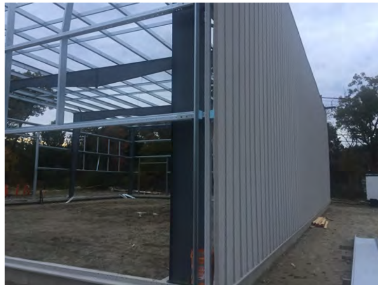
View of Panel wall
