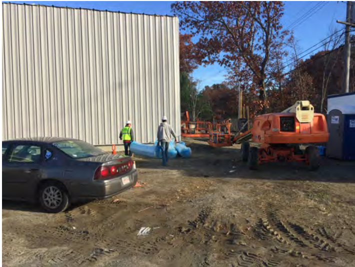
Crew prepping insulation for east wall panels
