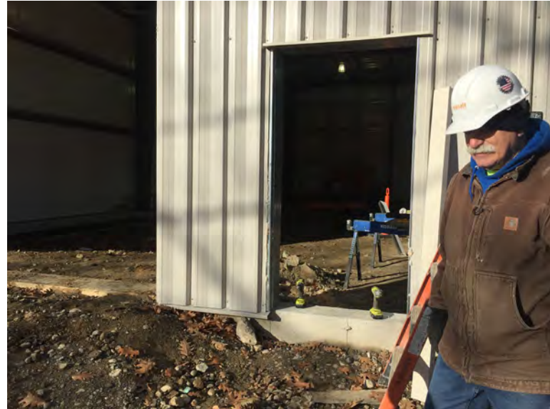
View prep work for man door installation
