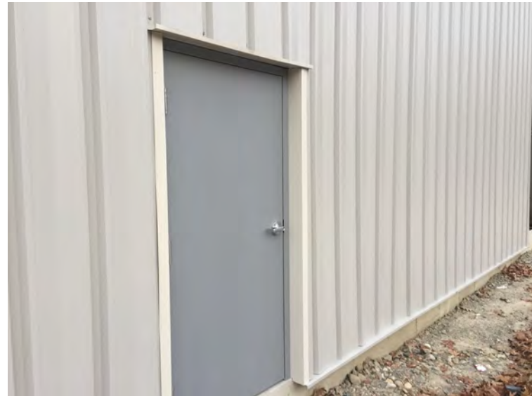
View of installed man door
