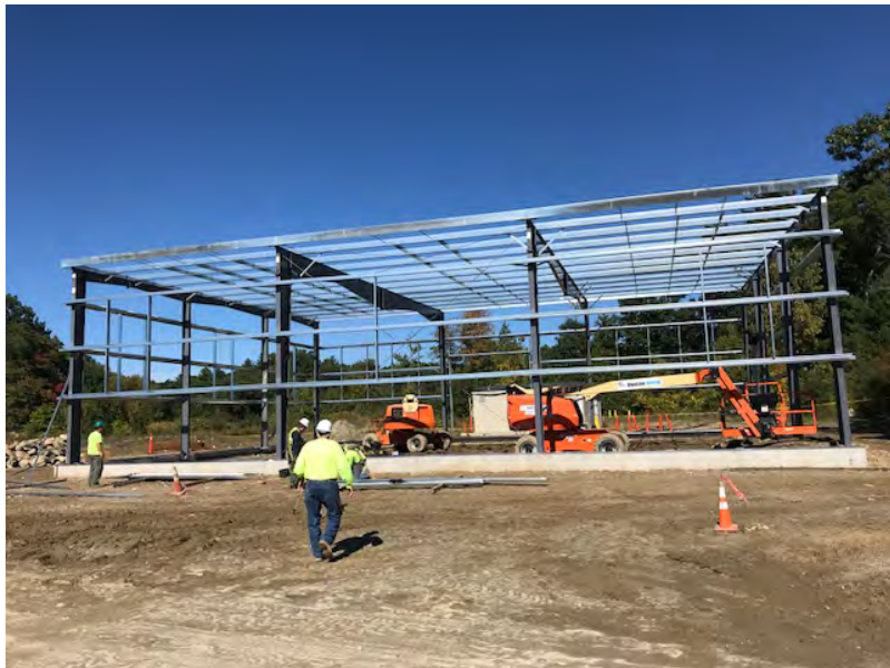
View of building progress
