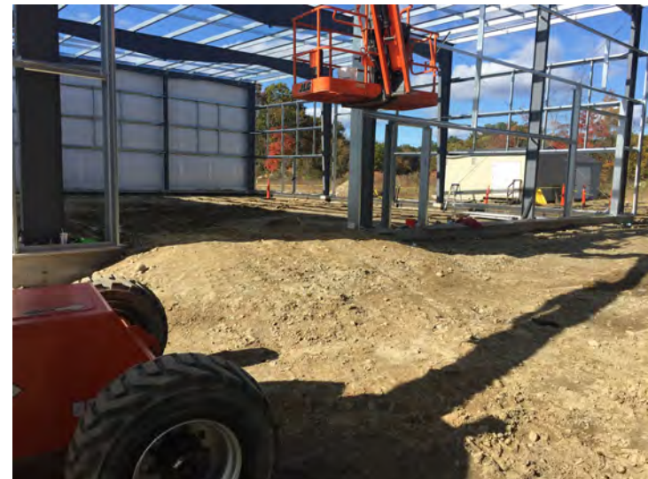
View of east wall with panel prep
