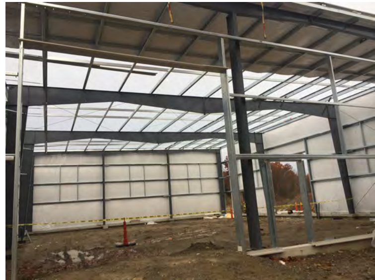
View of complete roof and wall work
