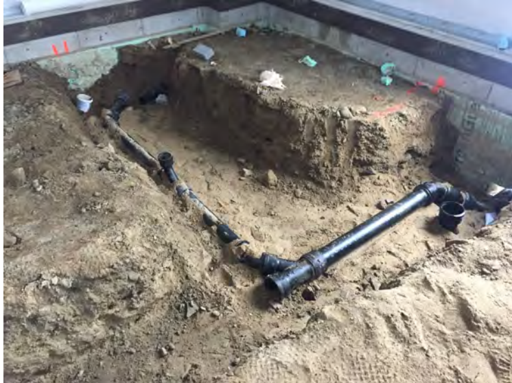
View of bathroom piping paced by plumber the day prior
