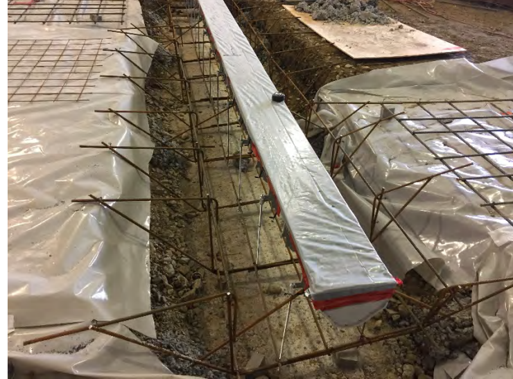
View of tied rebar in trench drain
