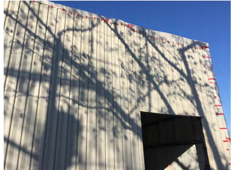
View of temporary trim on roof
