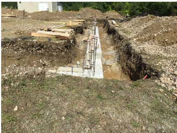
View of foundation with concrete solid
