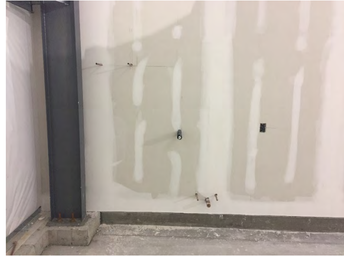
View of drywall on office
