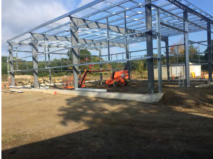
View of building interior structure
