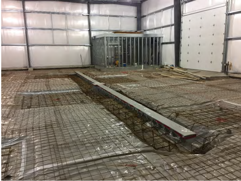
View of office framing
