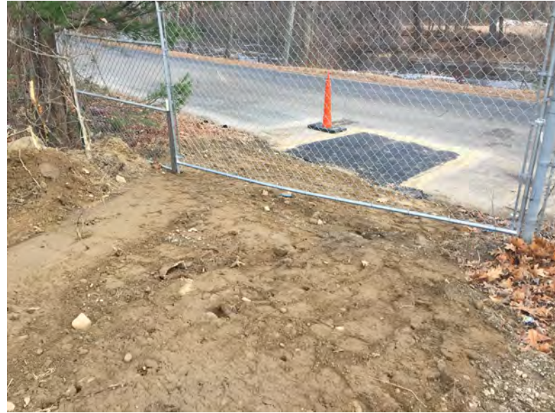
View of Onyx new asphalt and fence
