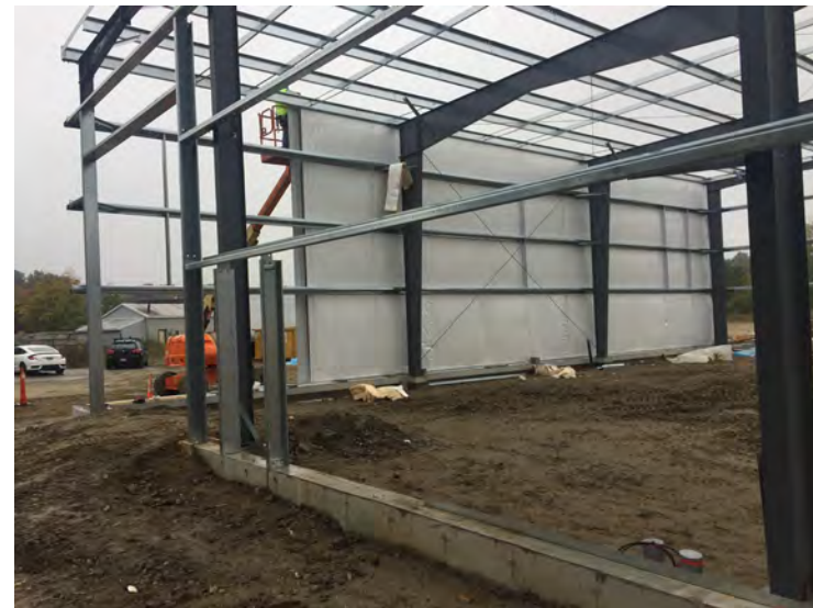
Inside view of insulation wall
