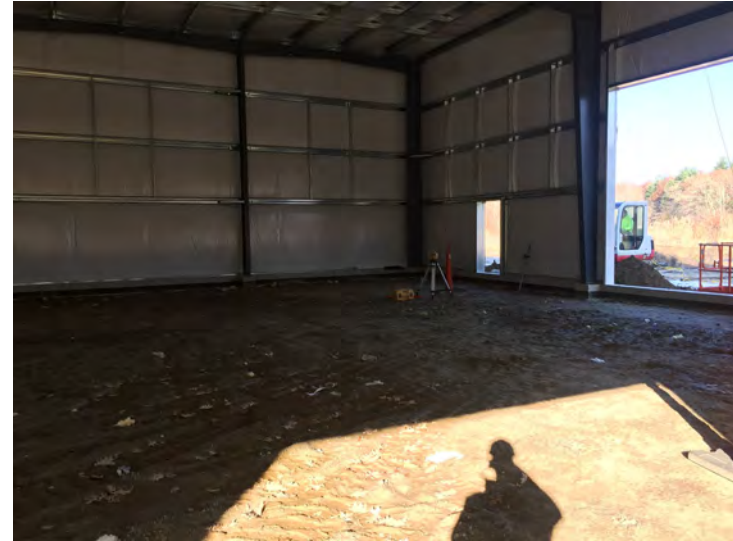
Prepping interior excavation work
