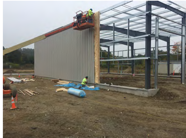
View of insulation, panel wall
