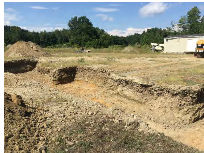
Part of the foundation dig completed
