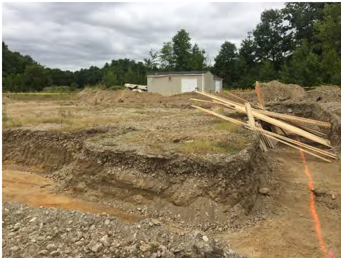
View of foundation hole with foundation lumber
