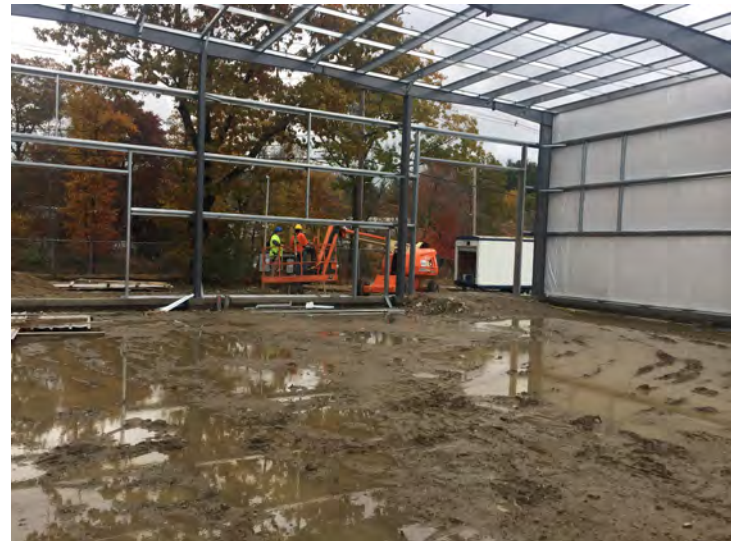
Working on panel walls
