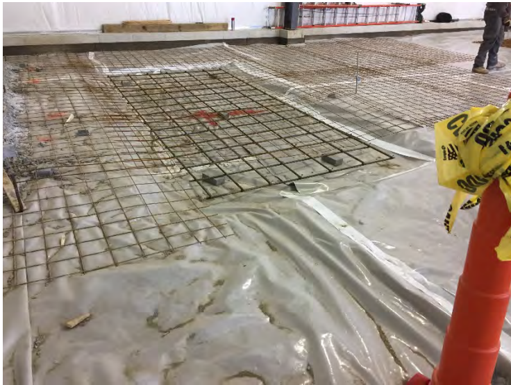
View of tied rebar
