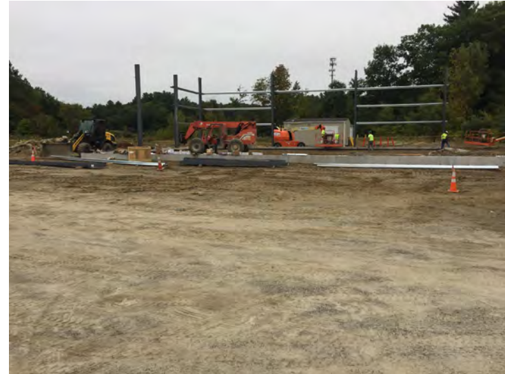
View building erection
