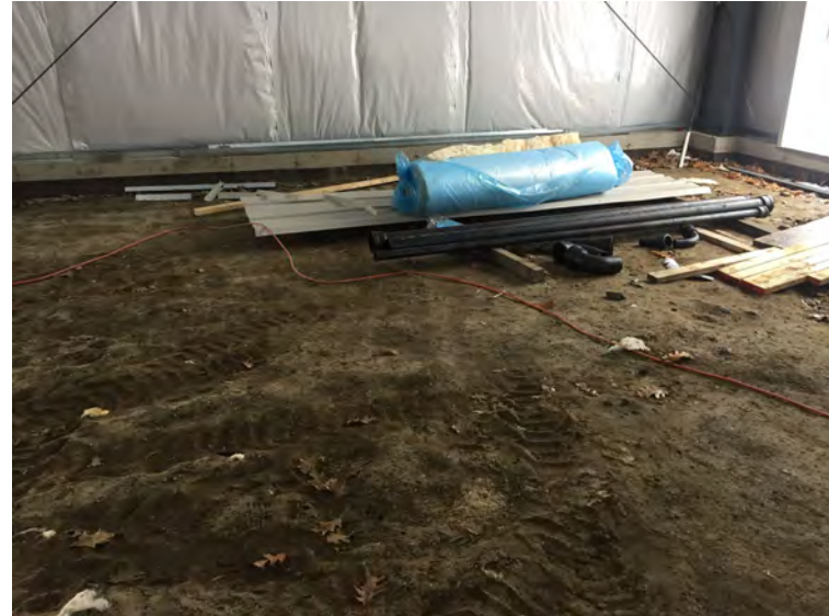
Pile of insulation, panels, trim, and piping inside building
