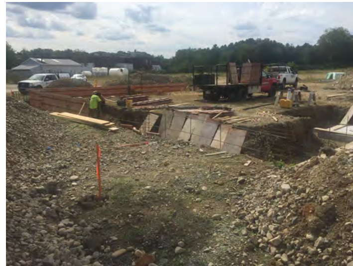
Samson placing concrete wall forms
