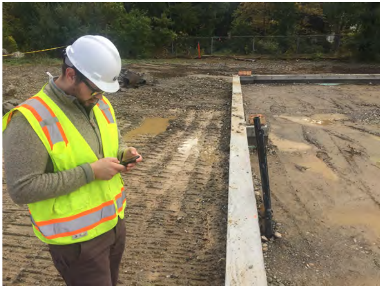
View of backfilled and compacted areas
