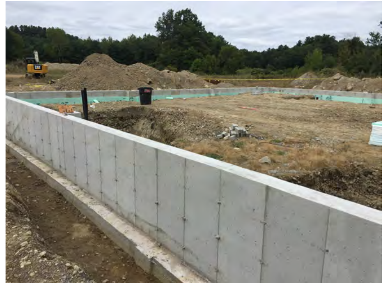
View of Foundation with insulation
