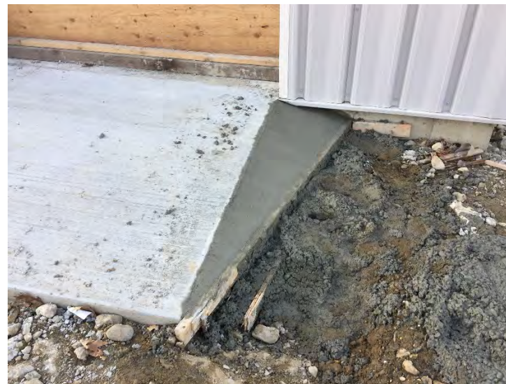
View of concrete work outside building
