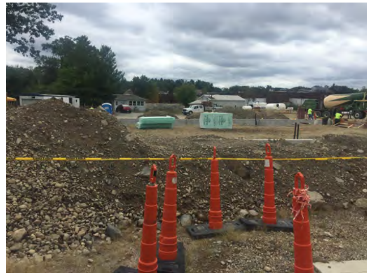
View of Site, concrete pour, and foundation insulation
