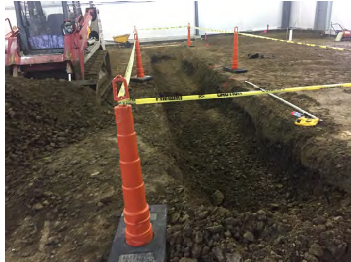
View of trench dug by Nashoba
