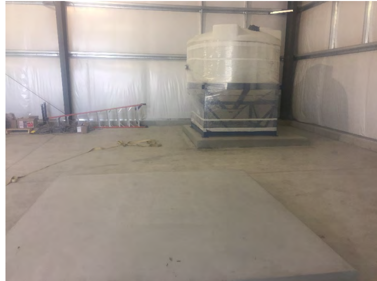
View of first tank placed
