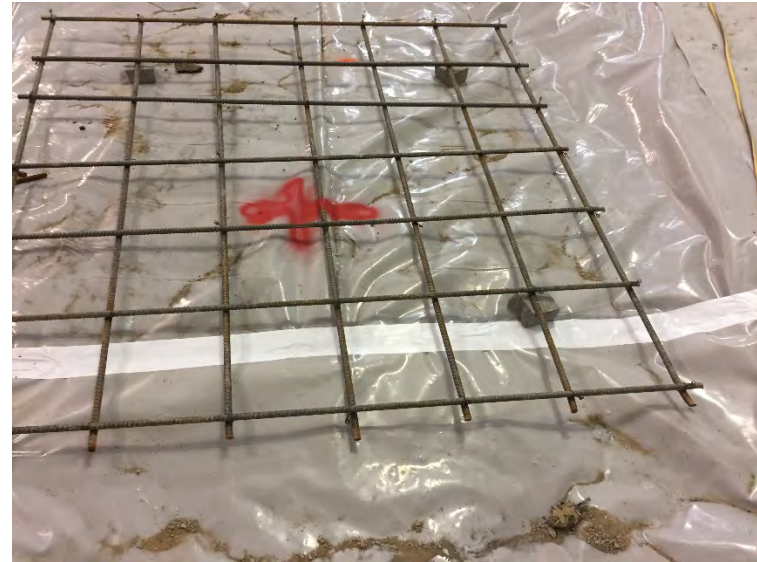
View of tied rebar
