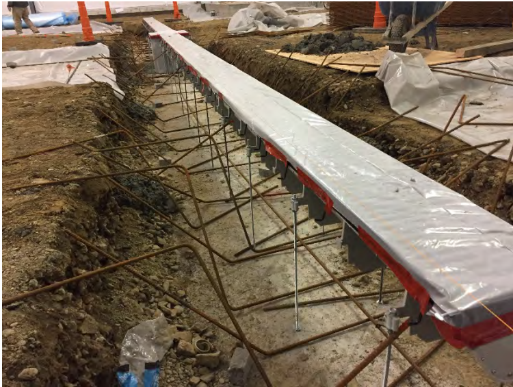
View of trench Drain supports
