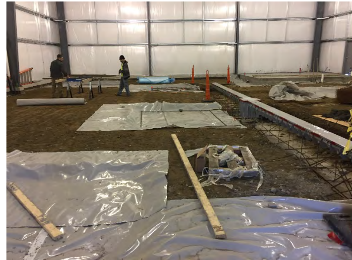
View of placing redar
