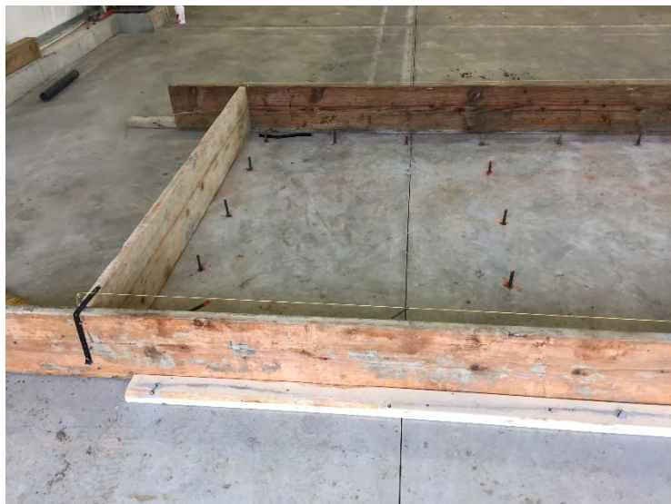
View of riser pad forms
