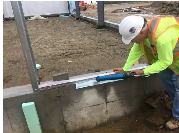
View of caulk being added to trim
