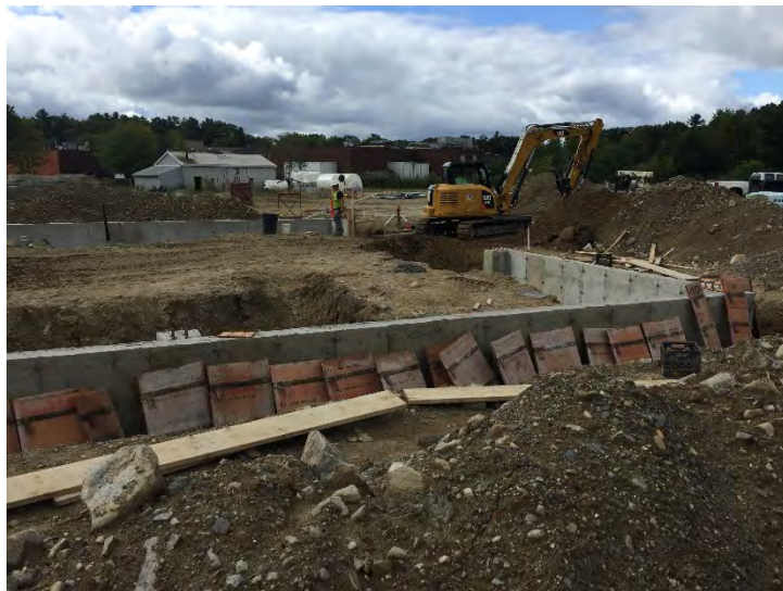
View of Nashoba digging final section of foundation
