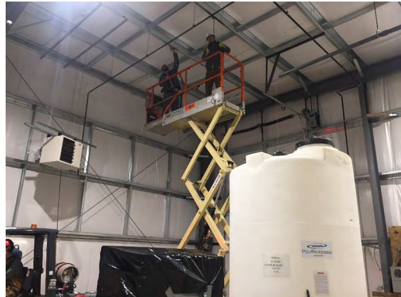
View of hanging pipe installation
