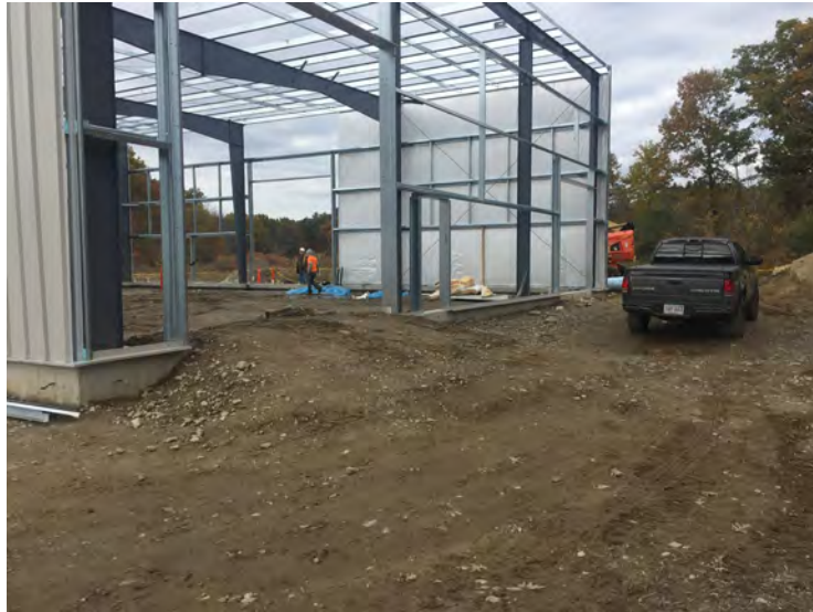
View of panels being placed
