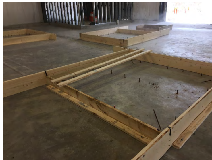
View of riser pad forms
