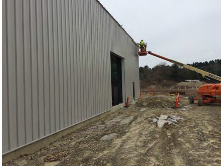
View of Regional placing roof trim
