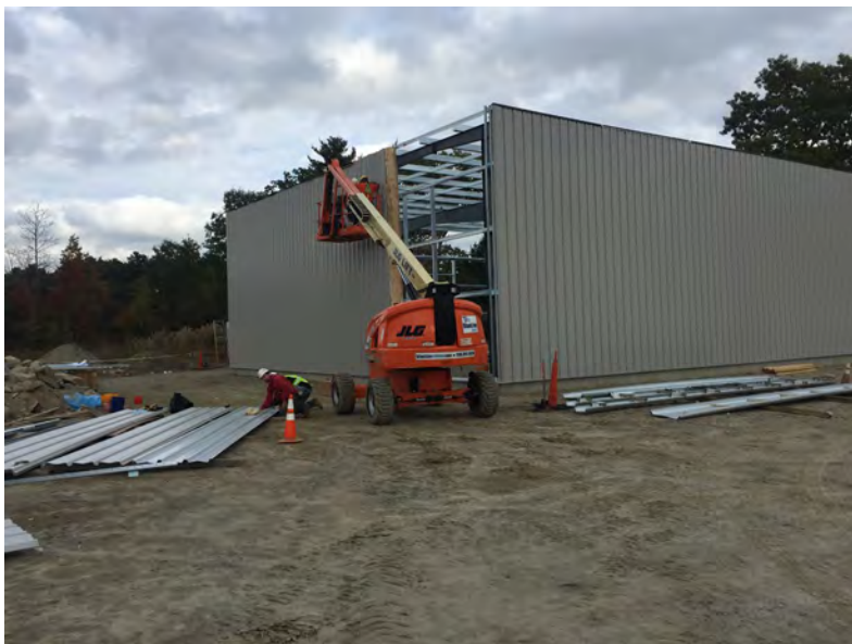
View of insulation/panels being placed
