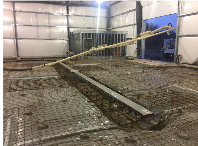
View concrete pump
