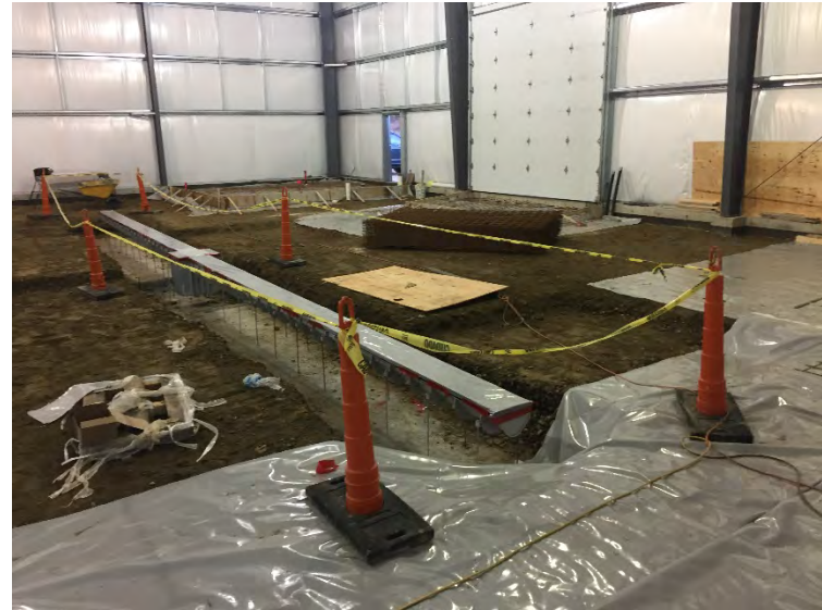
View of Concrete slab prep
