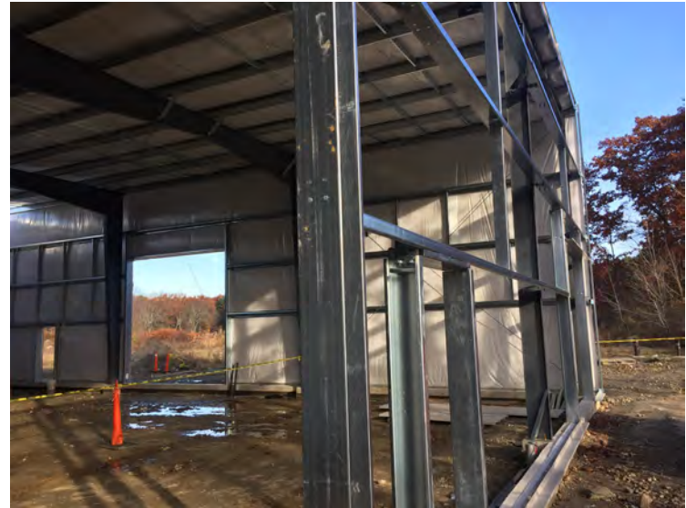
View of inside of building, and completed north wall
