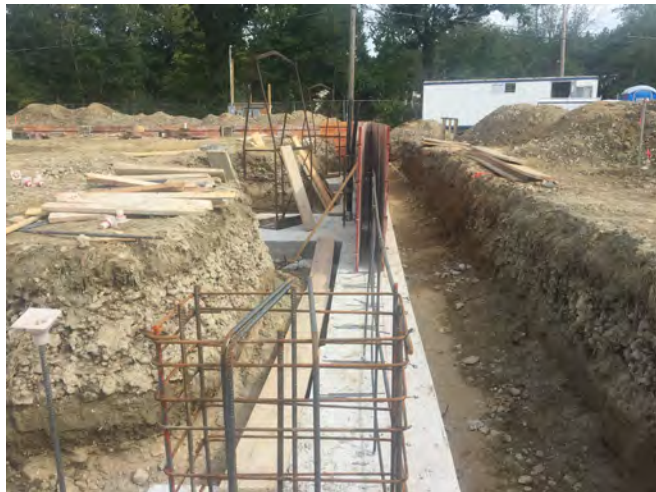
View of foundation wall forms
