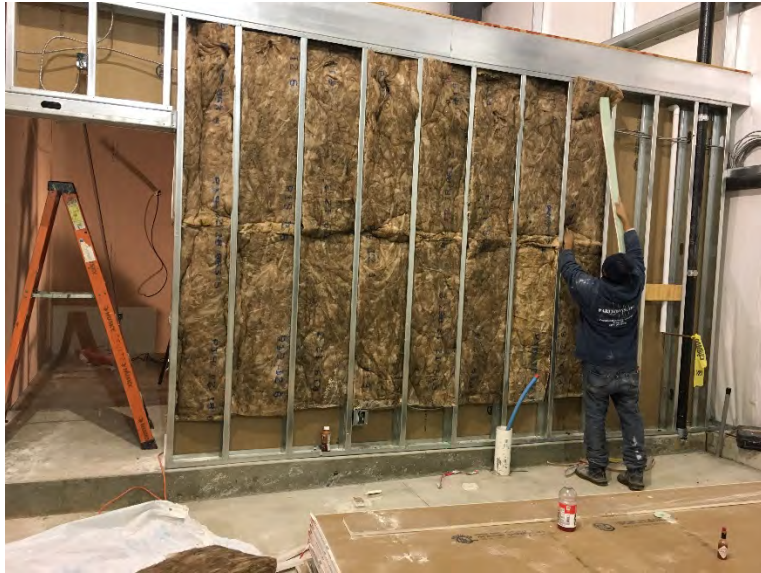
View of insulation in office walls
