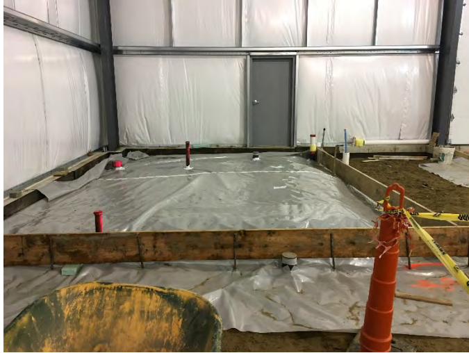
Framing of office slab
