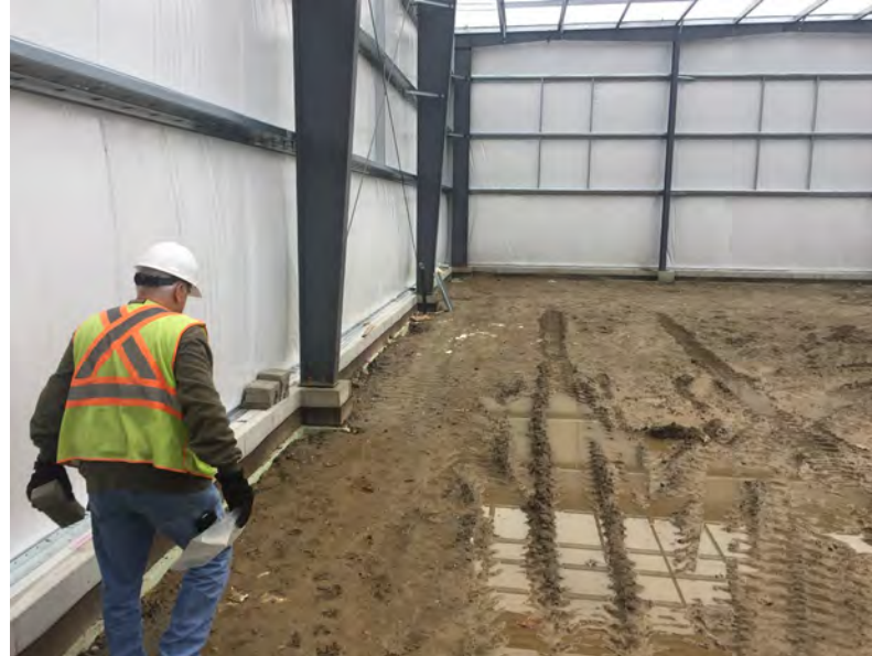
View of building corner
