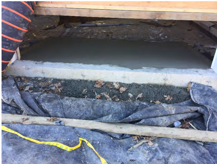
View of Concrete in ramp form
