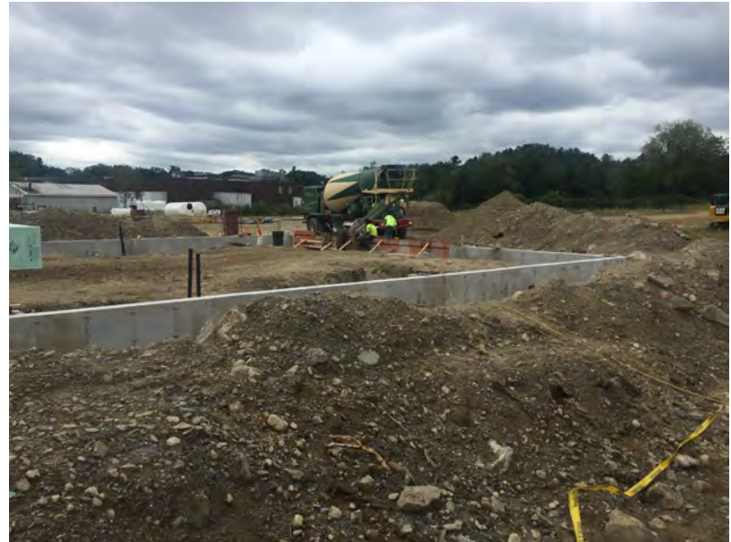
Concrete pouring of foundation wall
