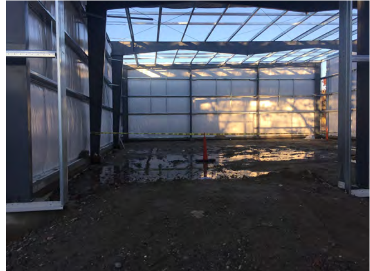
View of inside of building, and nearly completed north wall
