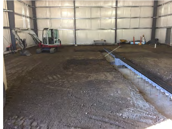
View of Grading work inside building
