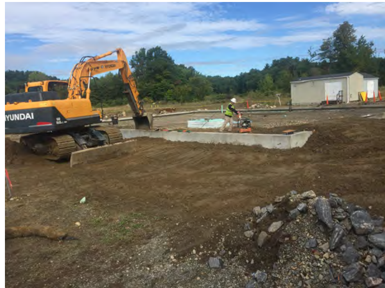
View of Nashoba backfilling and compacting around foundation
