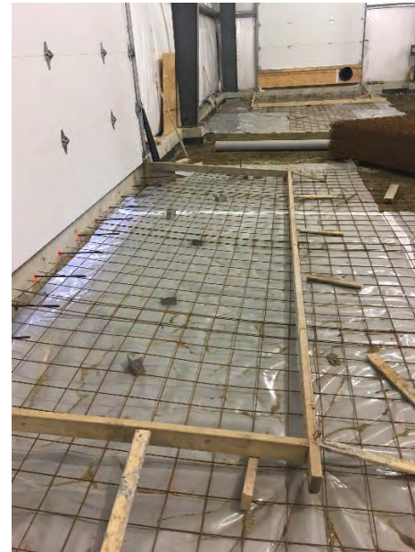
Mesh rebar in concrete ramp frames
