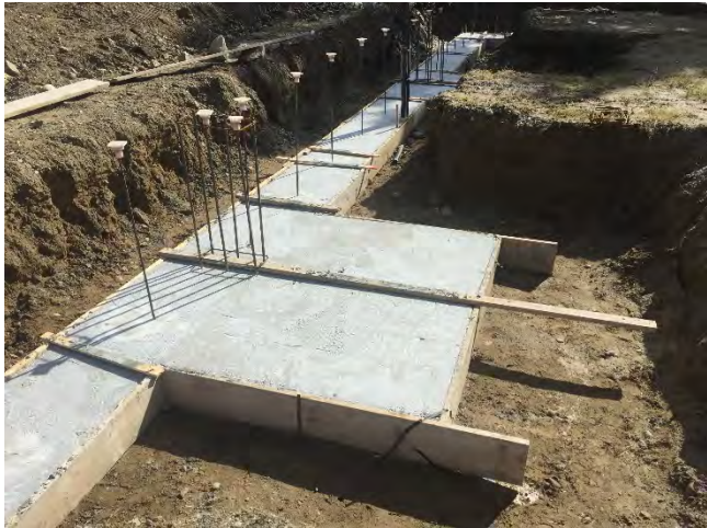
View of foundation with form still on
