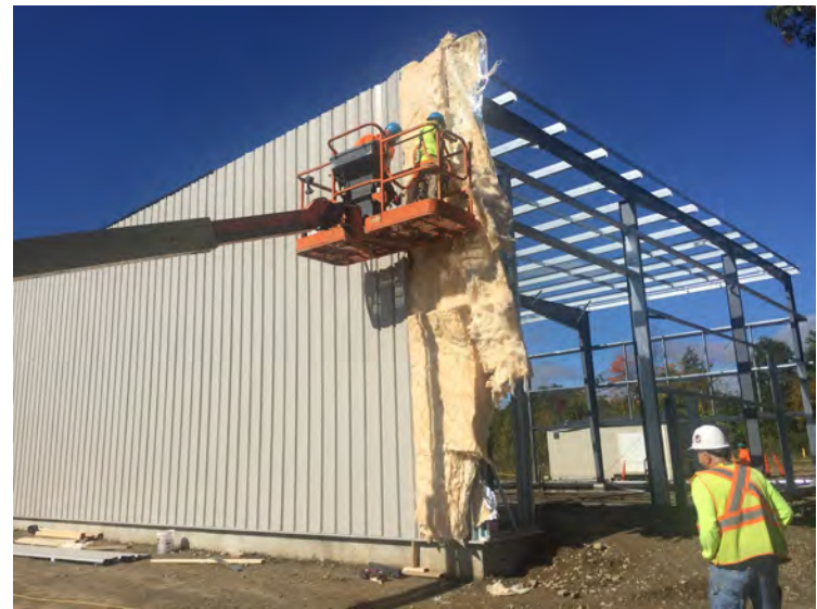
View of insulation, panel wall corner
