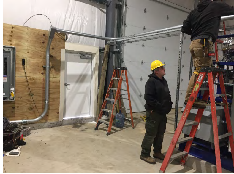
View of Watjus working on system electrical
