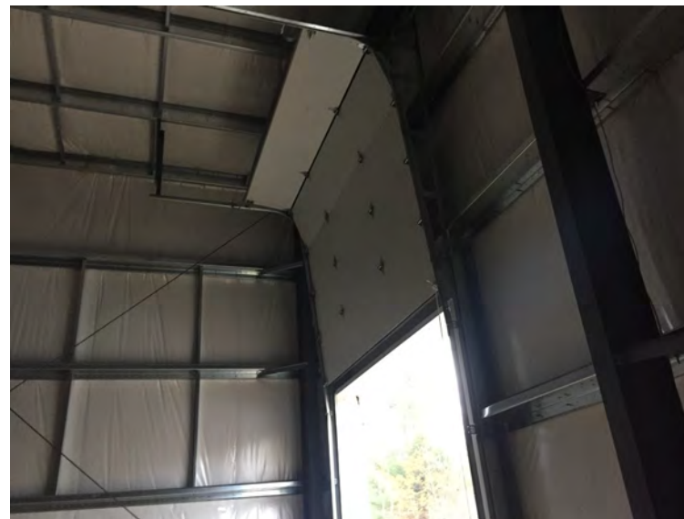
View of Frommelt building mechanical doors
