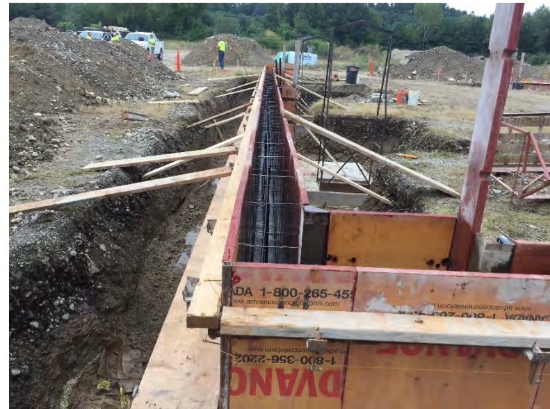
View of rebar in foundation wall forms
