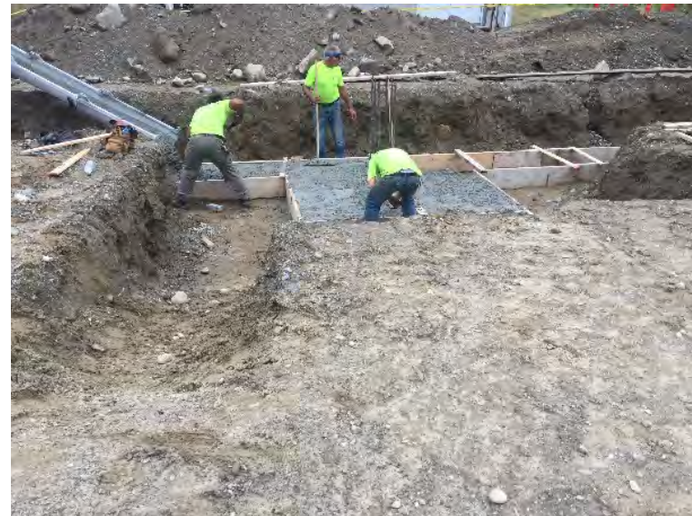
View of Samson placing concrete in foundation form
