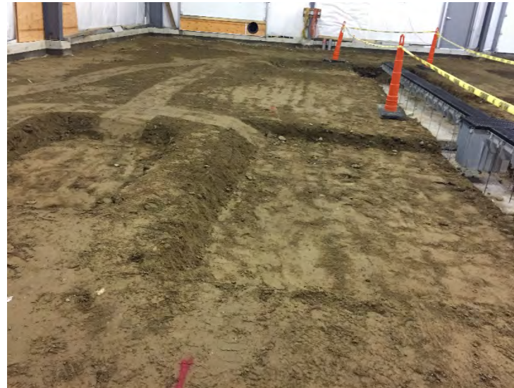
View of completed grading work
