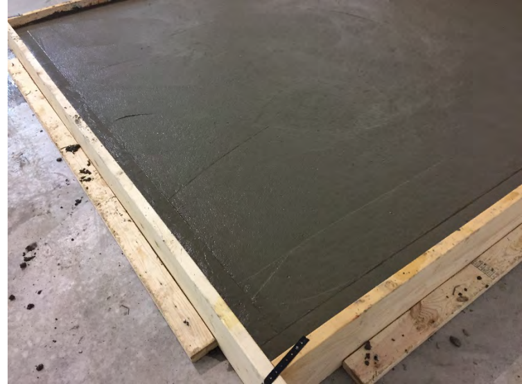
View of riser pad filled
