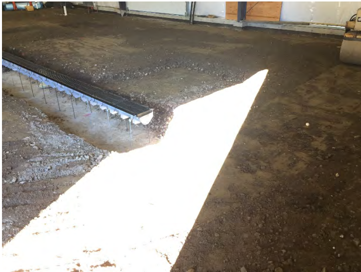
View of Grading work inside building
