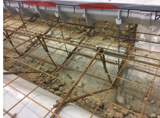
View of tied rebar in trench drain
