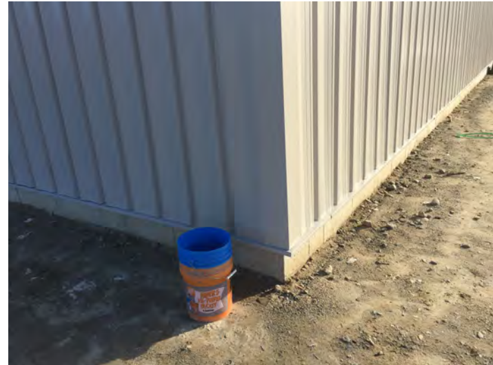
View of wall corner trim work
