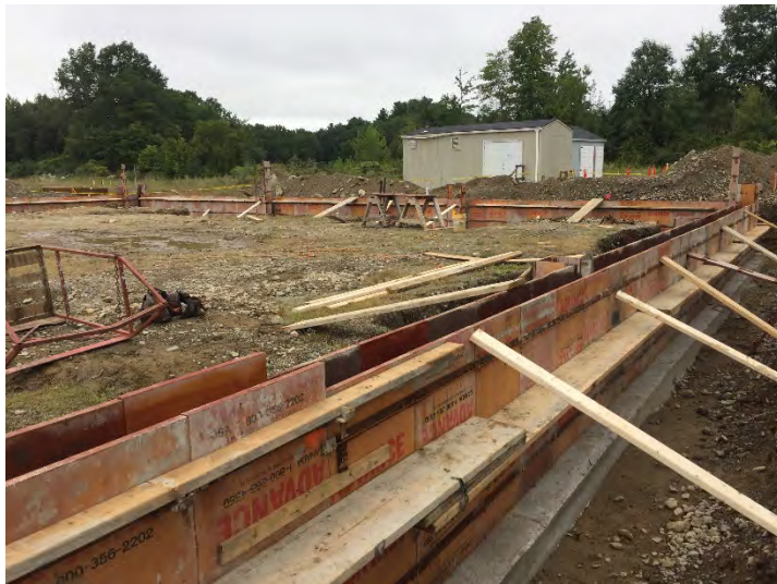
Final View of foundation wall forms
