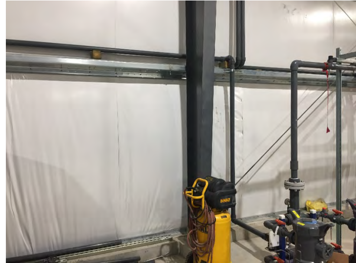
View of treatment system progress
