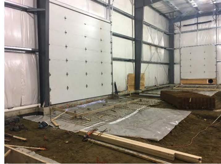
Mesh rebar in concrete ramp frames
