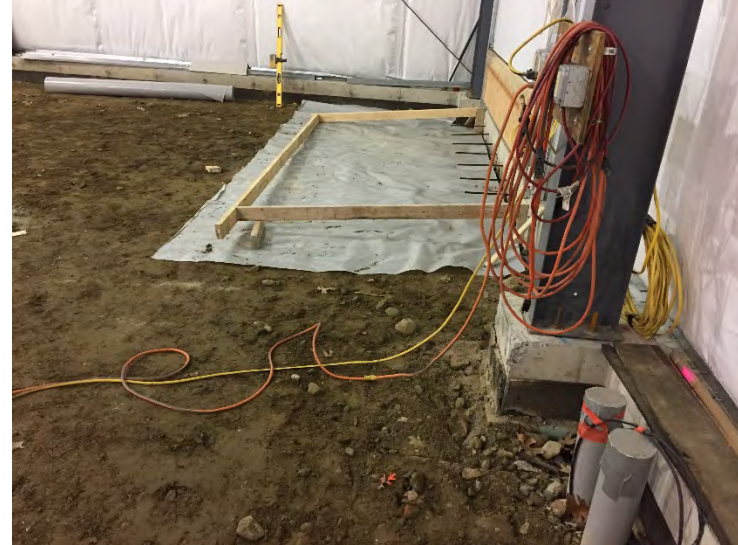
Framing of Door Ramps
