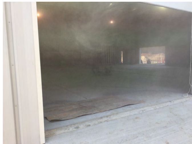
View of expansion joints being cut
