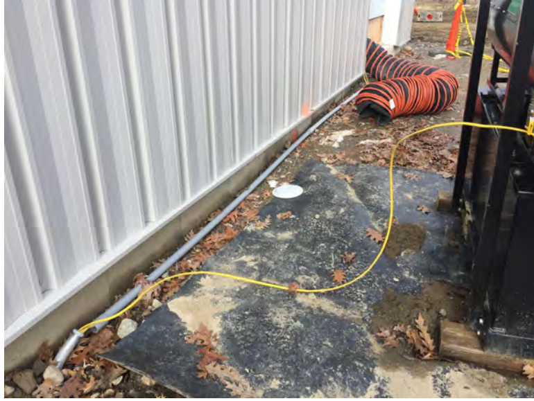
View of Electric work
