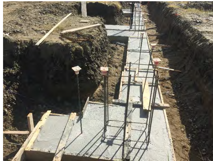
View of foundation with rebar
