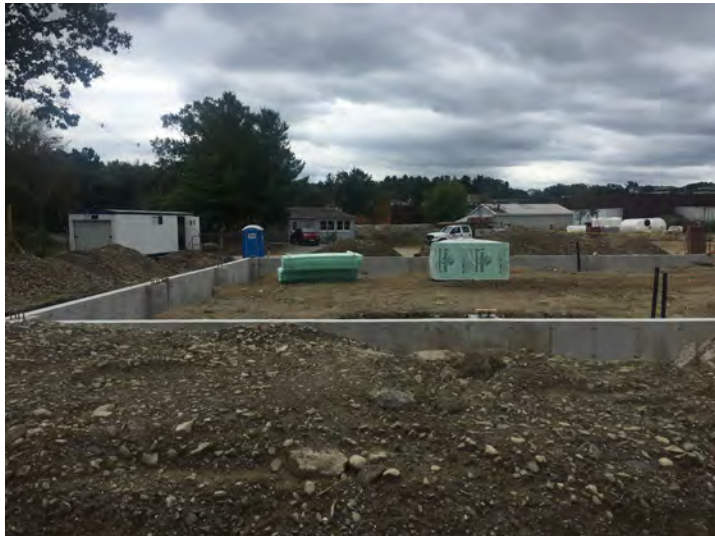
View of current foundation wall
