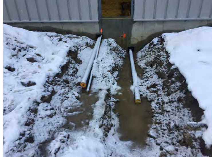
Underground plumbing for building office
