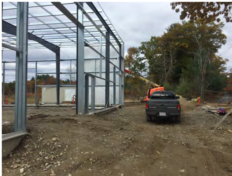
View of panels being placed
