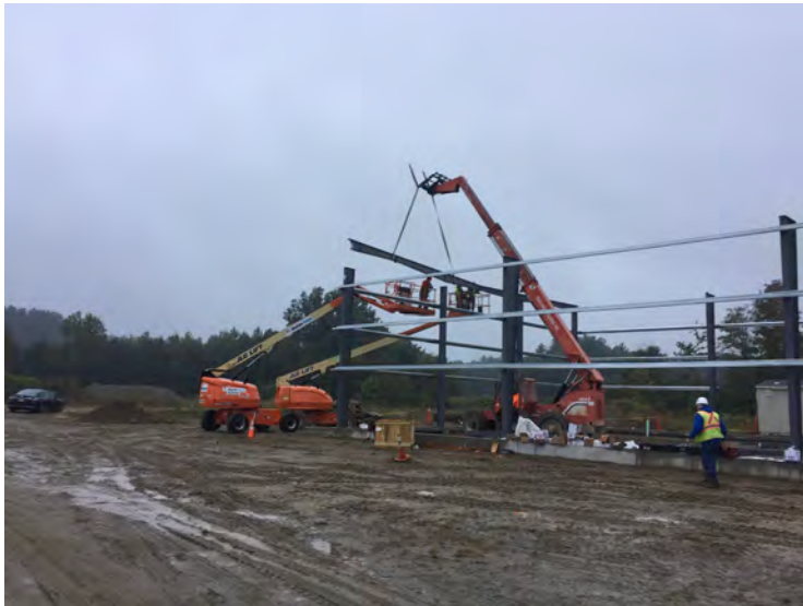
View builders continuing roof steel
