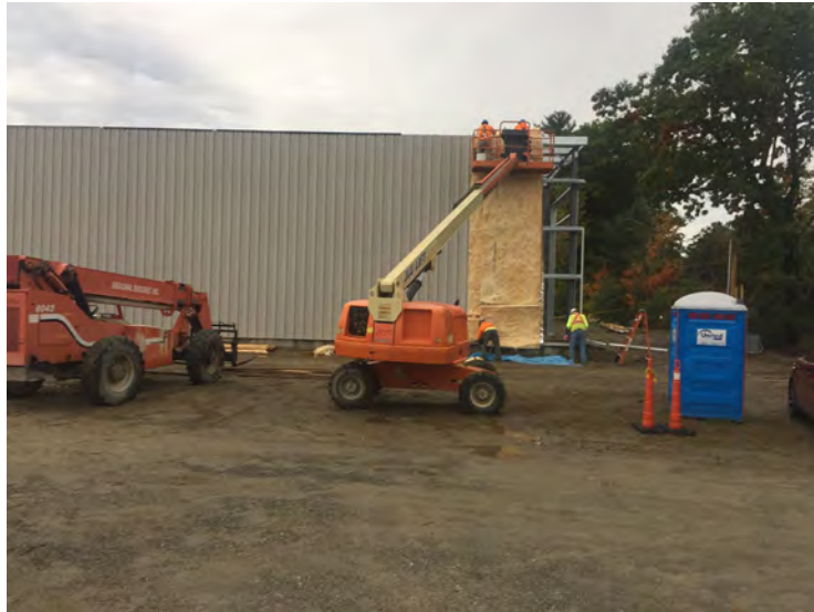
View of insulation, panel wall
