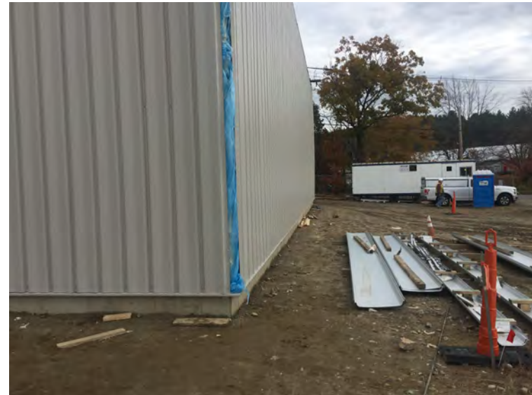
View of building corner
