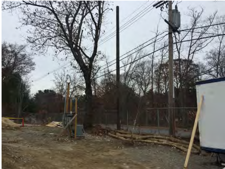
View of new telephone pole for permanent electricity
