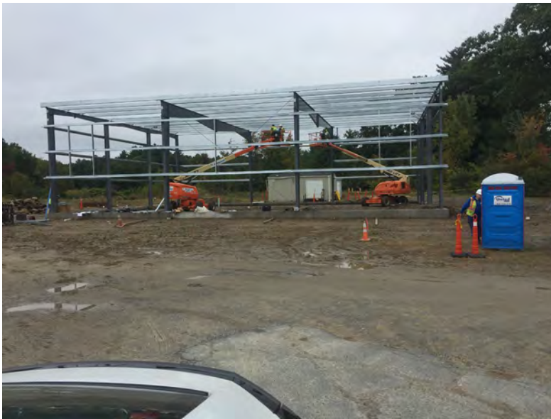
View of builders adding roof crossbeams
