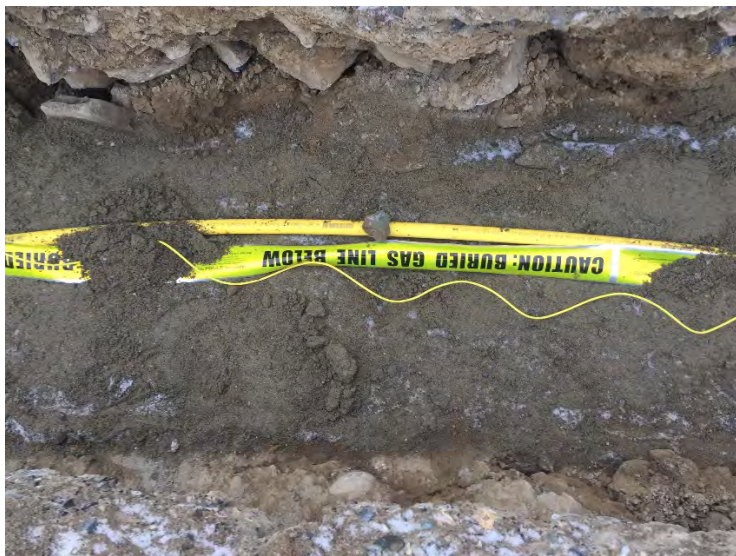
View of trench from propane tank to building
