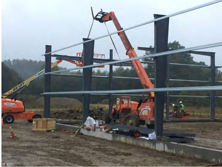
View builders starting roof steel
