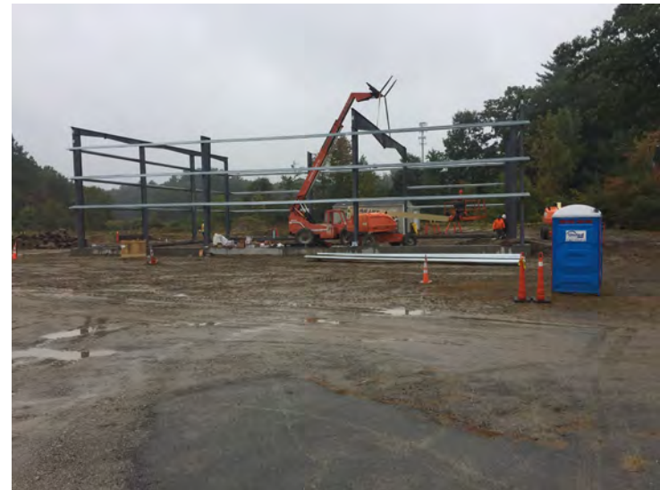
View builders continuing roof steel
