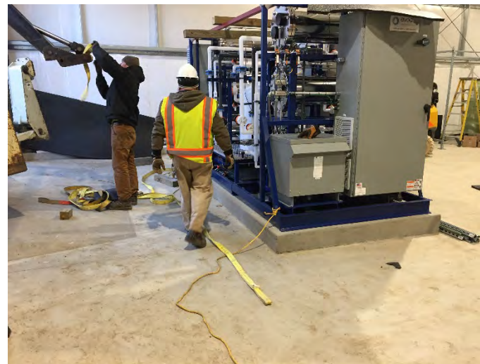
View of Vanox system bring brought into the building
