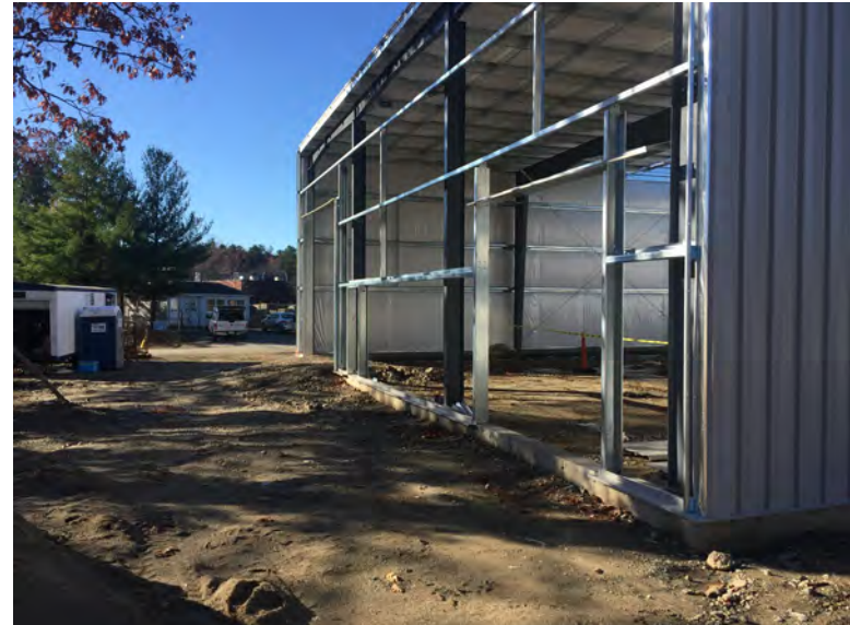
View East wall to begin being paneled tomorrow, 11/8/18
