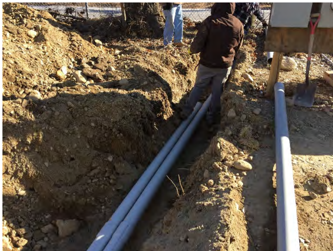
Electrician working on building wiring
