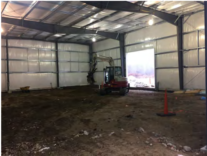
Nashoba filling in plumbing
