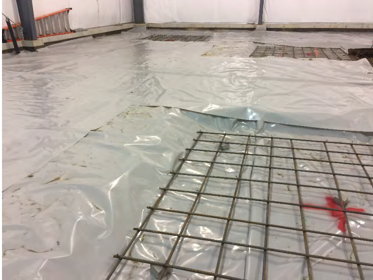
View of pad rebar
