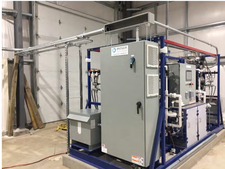
View of Electrical Layout for Vanox system
