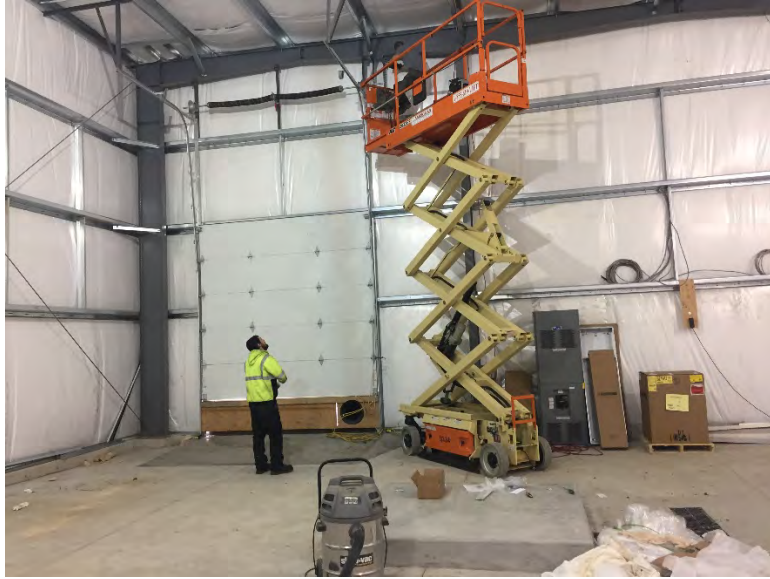
Frommelt attaching overhead door motors
