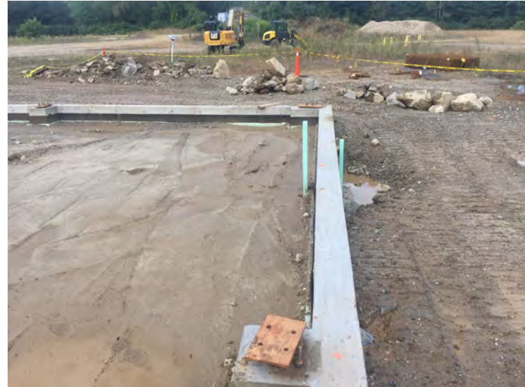
View of backfilled and compacted areas
