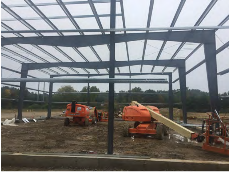
View building roof progress
