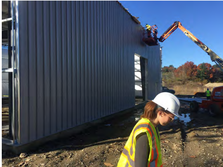
Crew working on north wall panels
