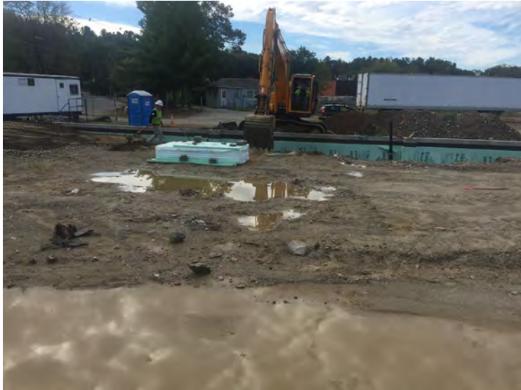
View contractors conducting backfill
