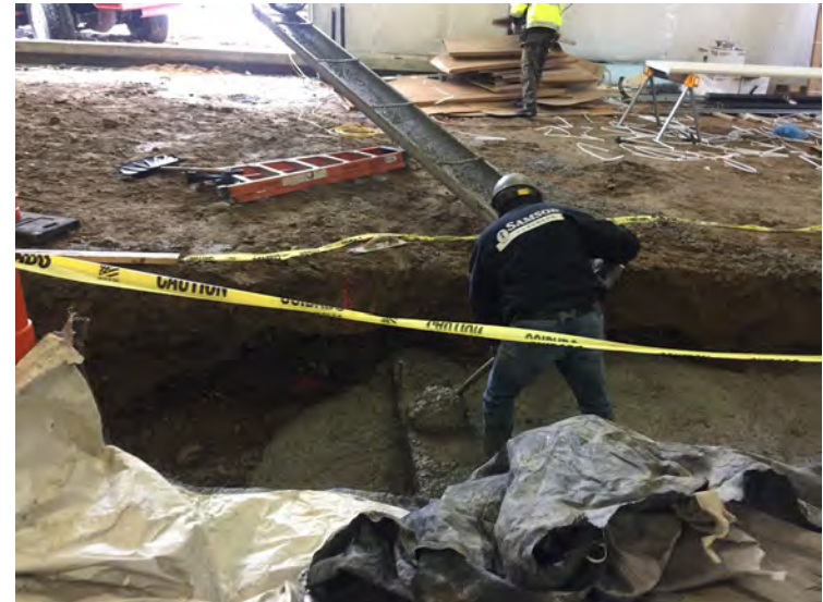
View of Samson Pouring concrete
