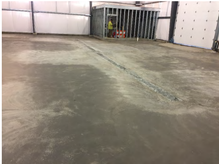
View of Concrete slab
