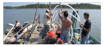
CMT Systems were installed at the bottom of a bay to measure submarine groundwater discharge. Eight 7-Channel CMT Systems were installed, with custom modifications to suit the open water application. Watertight wellheads had to be custom built to allow for sampling from the surface of the bay using a peristaltic pump.
